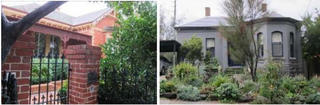
Two examples of the Victorian-era villas at 1 Yarra Grove & 3 Yarra Grove (Source: Context, 2017)
