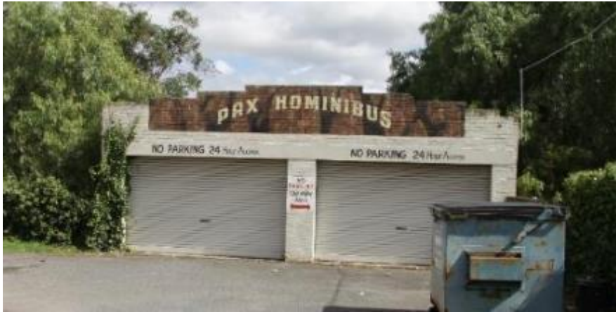
Figure 26. The double garage viewed from the east in the carpark, between the two peppercorn trees. (Source: Trethowan Architecture 2017)
