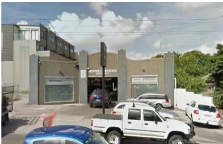
Figure 11. Motor garage, 878 Toorak Road, Hawthorn East (1920s). (Source: Google Maps 2017)
