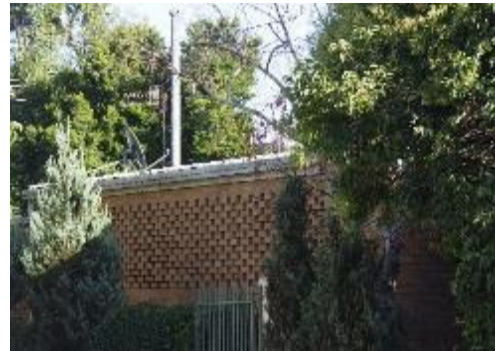
Figure 11. View of brickwork to rear of dwellings. Brickwork detail used as a filtered light source as per Figure 13. (Source: Trethowan Architecture, 2017)
