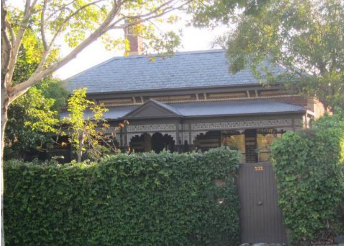
Figure 2. One of the three Victorian villas, at 202 Auburn Road. (Source: Context, 2017)
