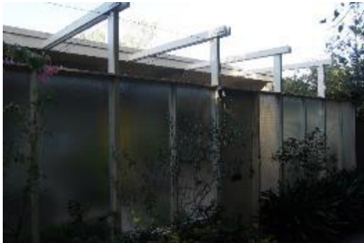
Figure 10. View of glazed partition wall to private courtyard. (Source: Trethowan Architecture, 2017)
