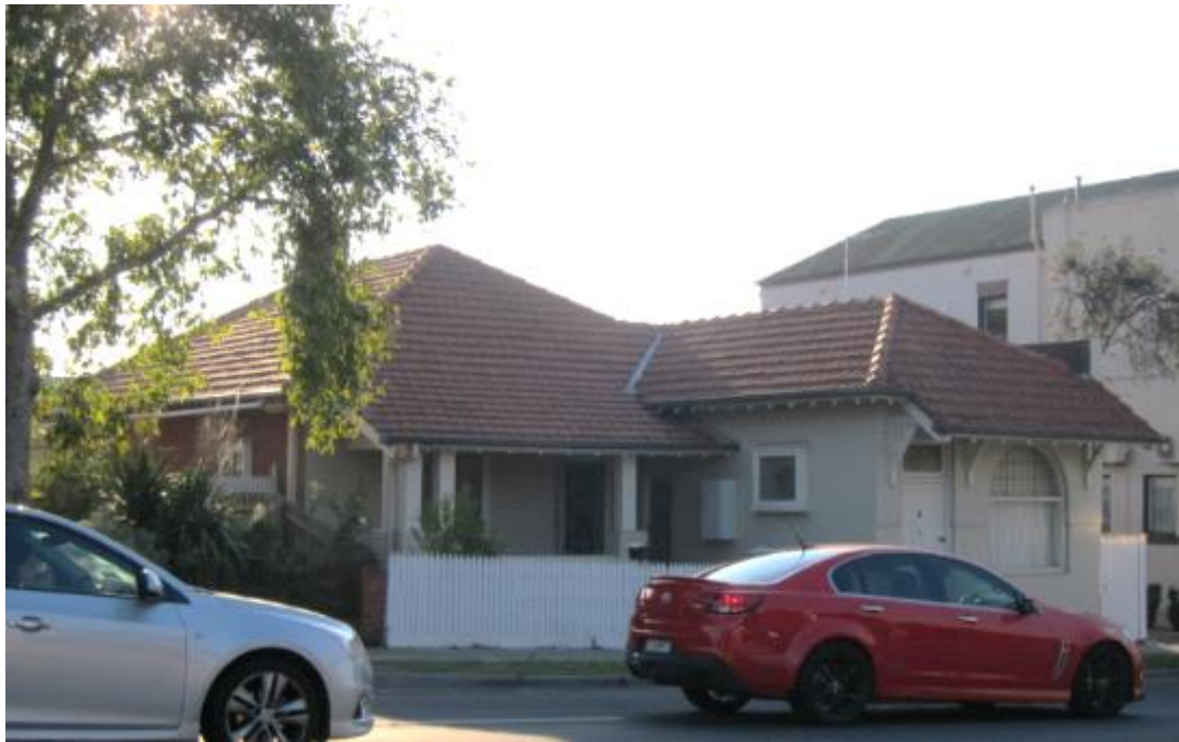
Figure 7. The bungalow with shop at the front, 172 Auburn Road. (Source: Context, 2017)
