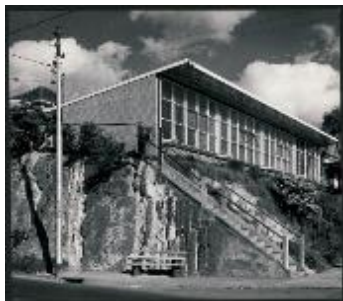
Figure 14. 'Bachelor flats', 2 Barkers Road, Hawthorn. Photograph by Wolfgang Sievers. (Source: State Library of Victoria)
