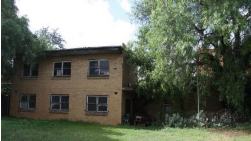
Figure 25. The post-war building attached to a garage, that may have been the c.1944 family home of the caretaker Romanin family. Beside it is a mature peppercorn tree from the original estate garden. (Source: Trethowan Architecture 2017)
