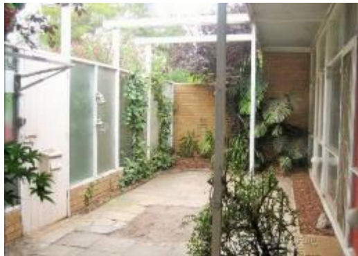
Figure 12. Private courtyard of Flat 1, looking east. Note the original timber door with inbuilt letterbox, square stone path, opaque glazed partition on raised brick wall and brick blade wall to separate courtyards. (Source: Realestate.com)
