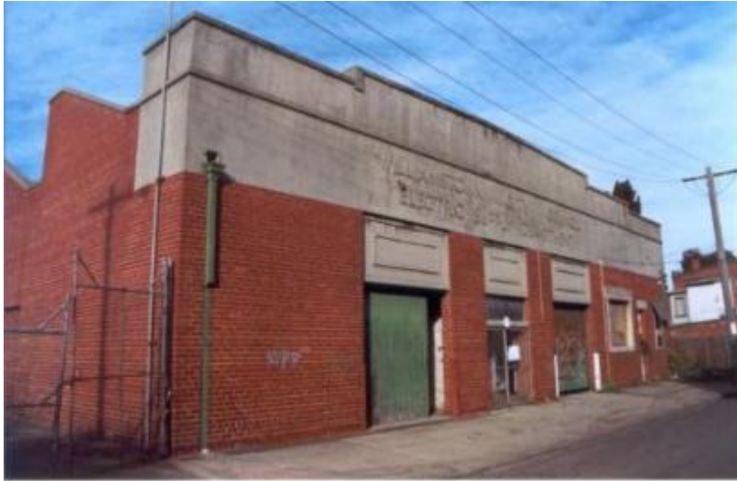
Figure 17. Williamstown City Council Electricity Supply Department (Former) 6 Bath Place Williamstown. (Source: Hobsons Bay City)
