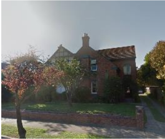
Figure 4. 'Berwyn Flats', 7 Glenroy Road. (Source: Google Maps, 2017)
