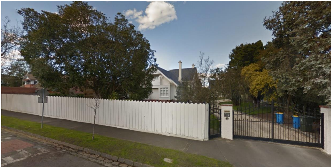
Figure 22. 12 Grange Road, Kew. (Source: Google Maps 2016)
