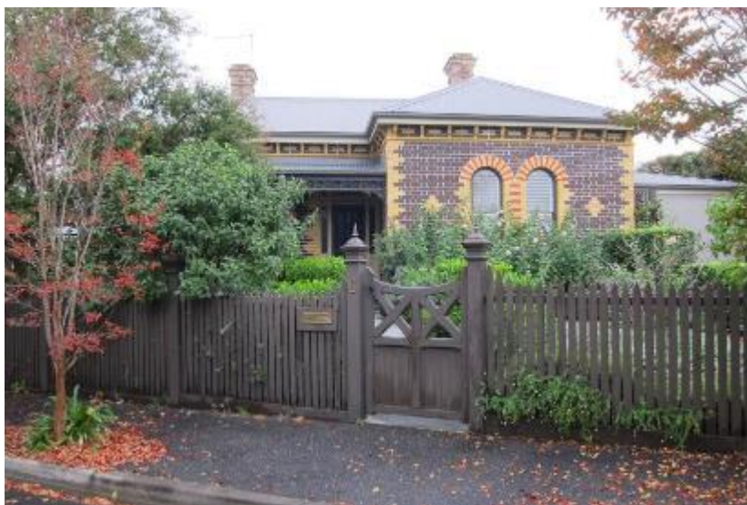
6 Austin Street, one of a pair with excellent polychrome brick patterning. (Source: context, 2017)
