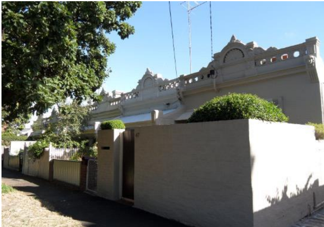
Figure 3. Single-storey late 1880s terrace at 37-47 Lennox Street. (Source: Context, 2017)
