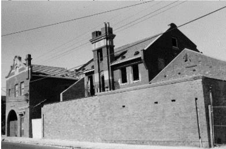
Figure 5. Farey Bro's Bakery, 1979. The photograph was taken during its conversion to offices. Note that the small gabled building behind the blank wall has been demolished with a gateway created at the east end, and two single chimneys behind it removed. (Source: SLV)
