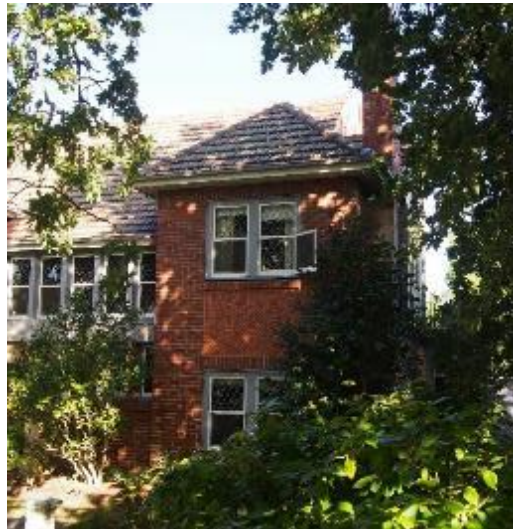
Figure 3. Northern aspect of street elevation. Note the diamond patterned glazing and tapestry brickwork applied in the band between the windows. (Source: Trethowan Architecture, 2017)
