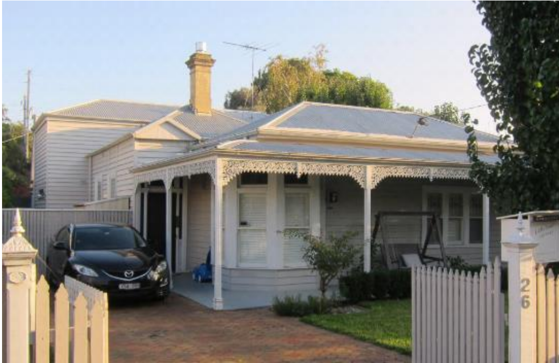
Figure 4. The early cottage (c1860s) at 26 Malmsbury Street. The front section with the very low hipped roof was built first, followed by the middle section with chimney (c1880s). The two-storey rear wing is recent. (Source: Context, 2017)
