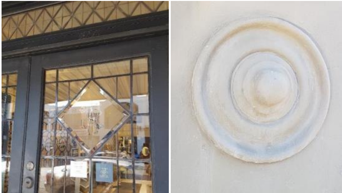
Figure 6. Detail of 'LRW' on diamond shaped glass panel in doors (left) and one of the cast wheel roundels on the piers (right). (Source: Trethowan 2017)
