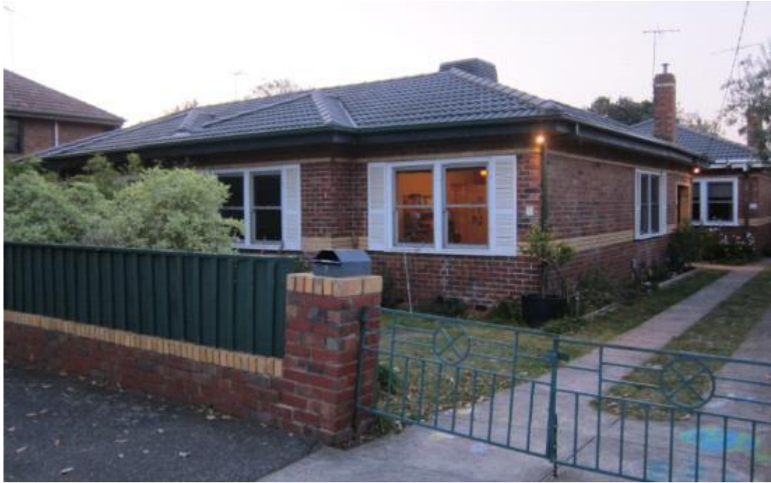
Figure 5. The flats at 5-7A Lennox Street, built c1935-38. Nos. 5 & 7 comprise the front semi-detached pair with Nos. 5A & 7A to the rear (No. 7A just visible at far right). (Source: Context, 2017)
