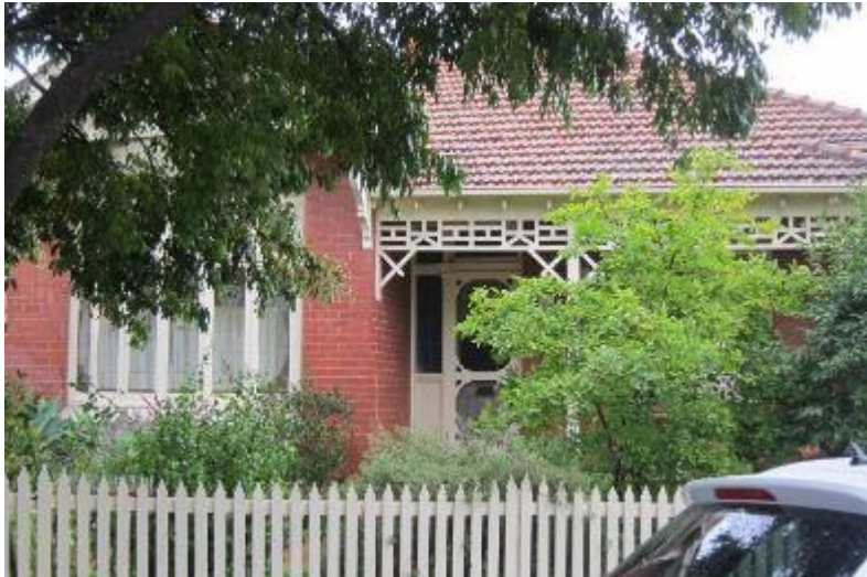
2 Manchester Street, a good example of a brick Federation house. (Source: Context, 2017)
