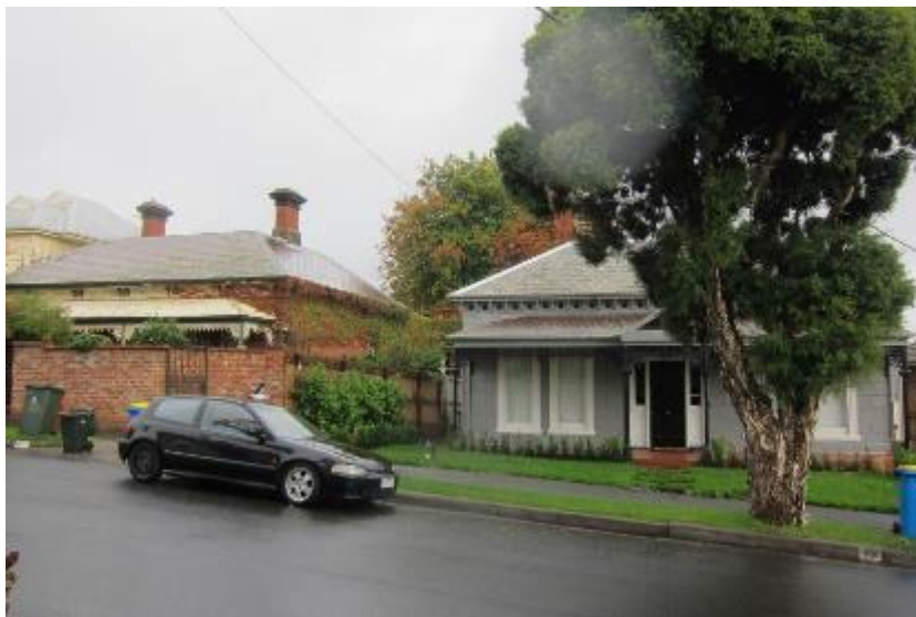
26 & 28 Illawarra Road, the precinct features both brick and timber Victorian villas. (Source: Context 2017)
