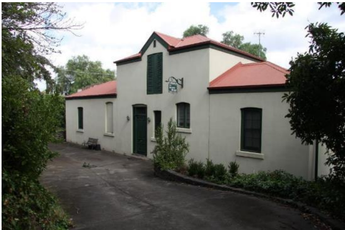
Figure 24. The stable block c.1903 is apparently all that remains of ‘Greystroke’, formerly 122 Power Street. (Source: Trethowan Architecture 2017)
