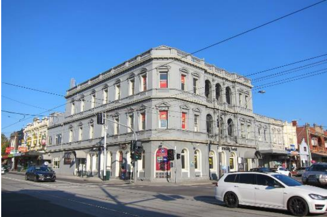
Figure 1. Three-storey Italianate style corner hotel at 277 Auburn Road (HO595), flanked by Victorian, Edwardian and interwar shops lining Riversdale and Auburn roads. Visible at the far right of the image is the individually significant W.A. Carr's Butcher Shop (HO596). (Source: Context)
