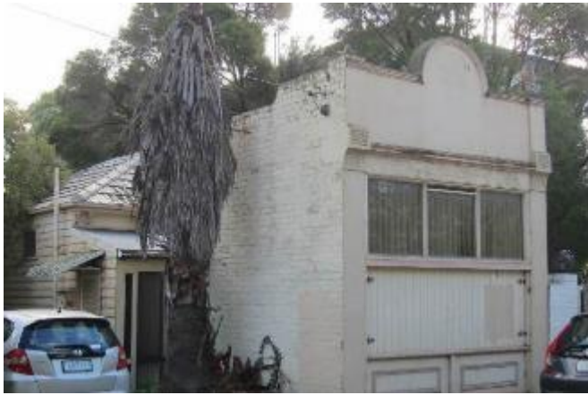
Shop and a palm tree at 48 Bell Street. (Source: Context, 2017)
