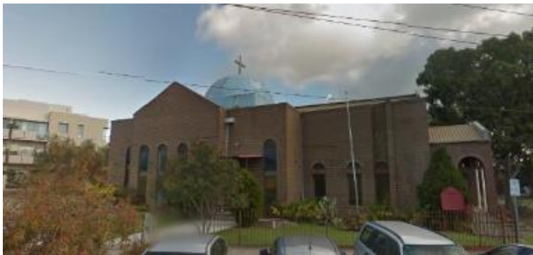
Figure 33. Greek Orthodox Chapel, 15 Rose Street, Hawthorn East. (Source: Google Maps)
