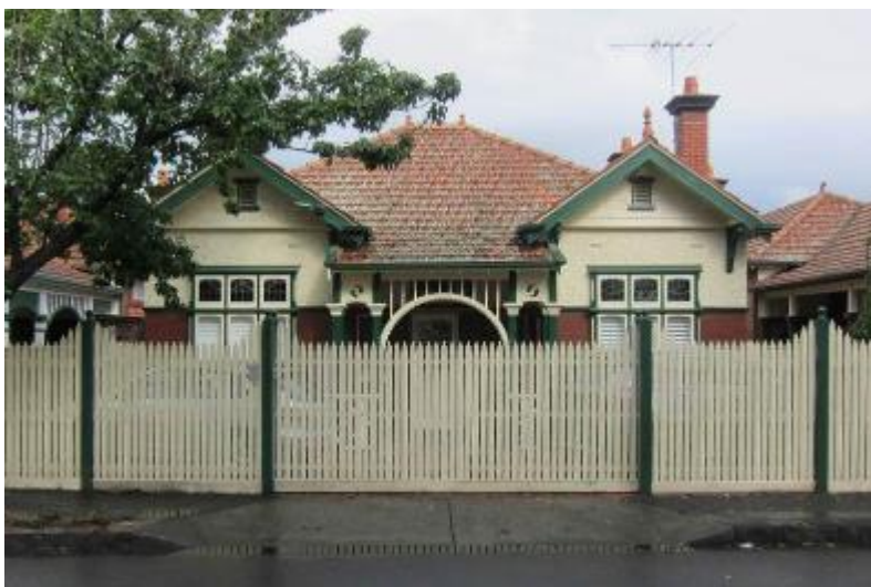
The central house, no.100 between 96-98 and 102-104 Liddiard Street. (Source: Context, 2017)
