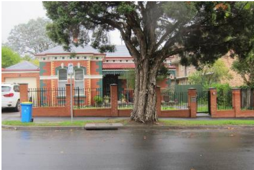
10 Illawarra Road, may be compared with 7 Illawarra Road in the brick quoins and box bay window. (Source: Context, 2017)
