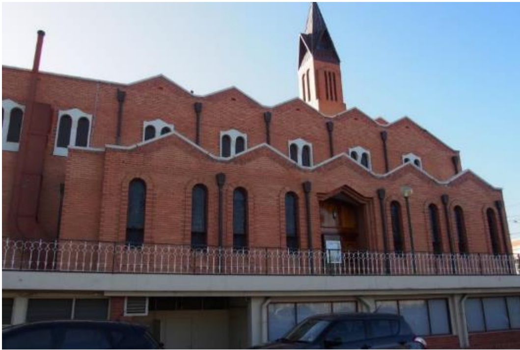
Figure 16. Eastern façade of the church showing regular parapet pattern, brick relief doorway into the gallery, arched stained glass gallery windows, and paired concrete-framed clerestory windows. Basement rooms open onto the car park. (Source: Trethowan Architecture 2017)
