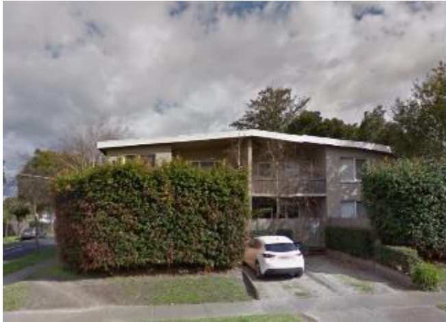
Figure 8. Flats, 157 Highfield Road, Camberwell (1960) designed by Peter McIntyre. (Source: Google Maps)
