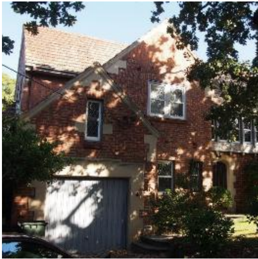
Figure 2. Southern aspect of street elevation including front garage. Note the tapestry brickwork applied in the gable and quoining details. (Source: Trethowan Architecture, 2017)
