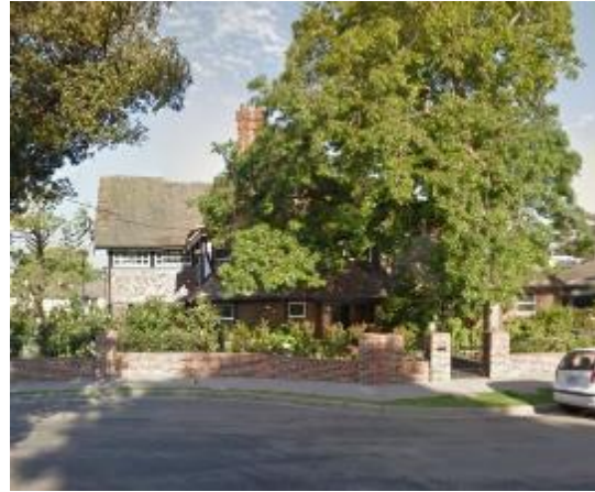
Figure 5. 2 Daracombe Road. (Source: Google Maps, 2017)
