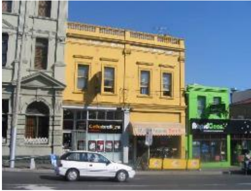
Pair of Victorian shops at 344-346 Burwood Road, Hawthorn. (Source Context, 2009) Included as a Contributory place in HO491. One shopfront with a splayed and recessed entry and the other replaced entirely.
