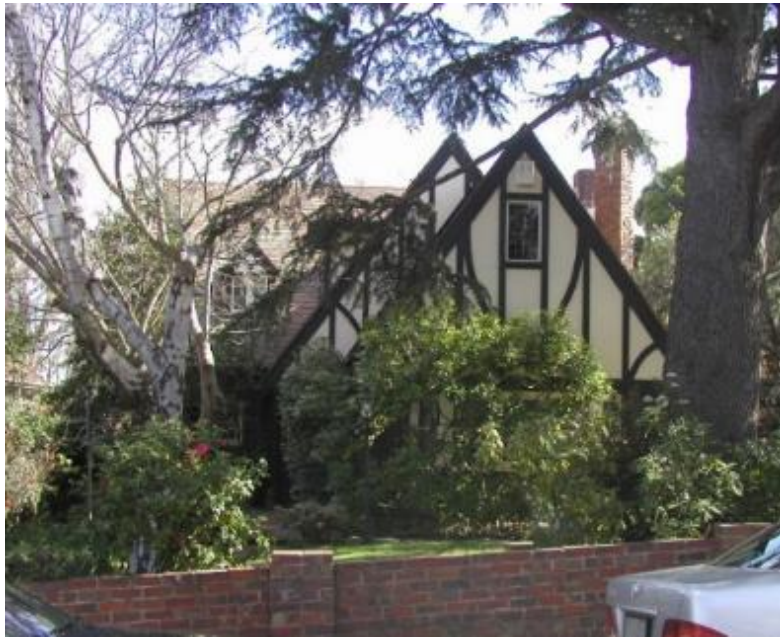
Figure 6. View of 19 Howard Street, Kew. (Source: City of Boroondara HO528)
