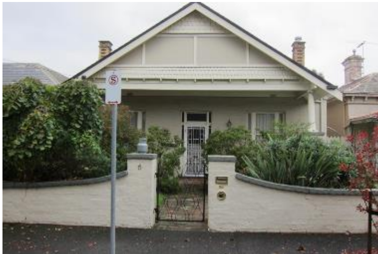
6 Majore Street, altered 1877-1879 house. (Source: Context, 2017)
