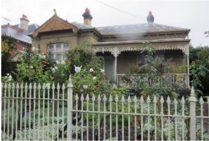
24 Robinson Road, a Victorian/Federation house transitional with features that are transitional. | (Source: Context, 2017)
