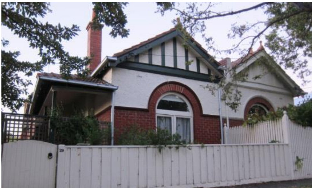
Figure 4. Edwardian semi-detached dwellings at 29-31 Lennox Street. (Source: Context, 2017)
