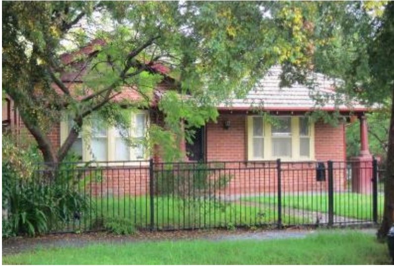
22 Violet Grove, an Interwar bungalow that is atypical in the precinct. (Source: Context, 2017)
