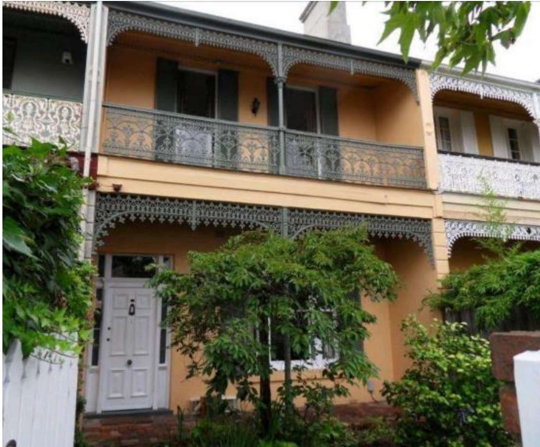
Figure 3. 213 Auburn Road, showing the front door. (Source: Realestateview.com, nd)
