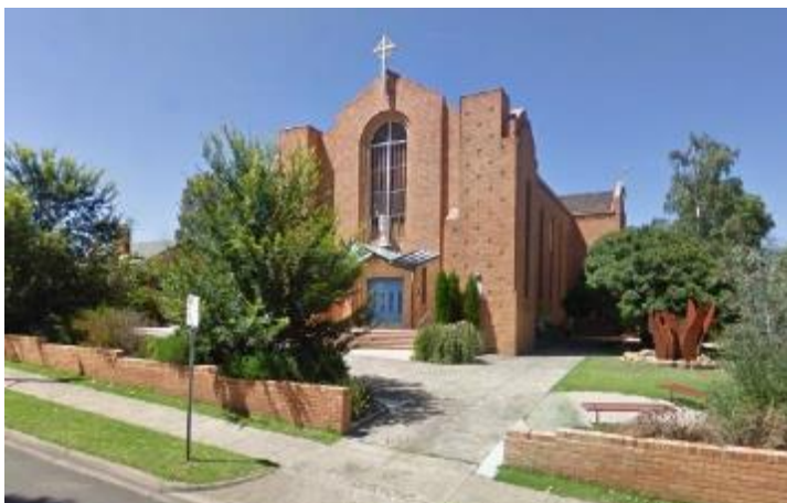
Figure 30. St Michael's Ashburton. (Source: Google Maps)
