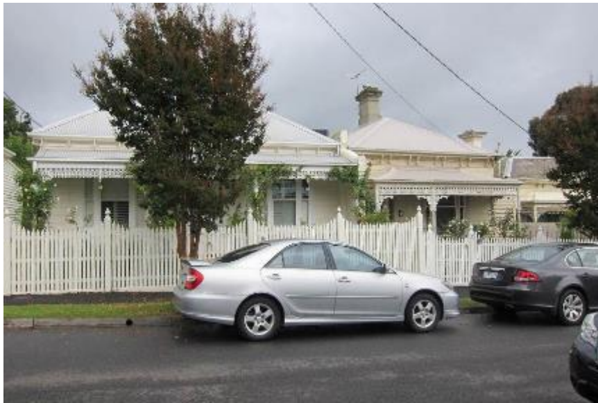
Violet Grove, typical Victorian-era timber residences. (Source: Context, 2017)
