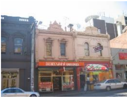
Victorian shops at 355-361 Burwood road Hawthorn, (Source: Context, 2009) Included as a Contributory place in HO491. Different pediments used to distinguish each building and some high quality moulded stucco around the windows on the left-hand shop.
