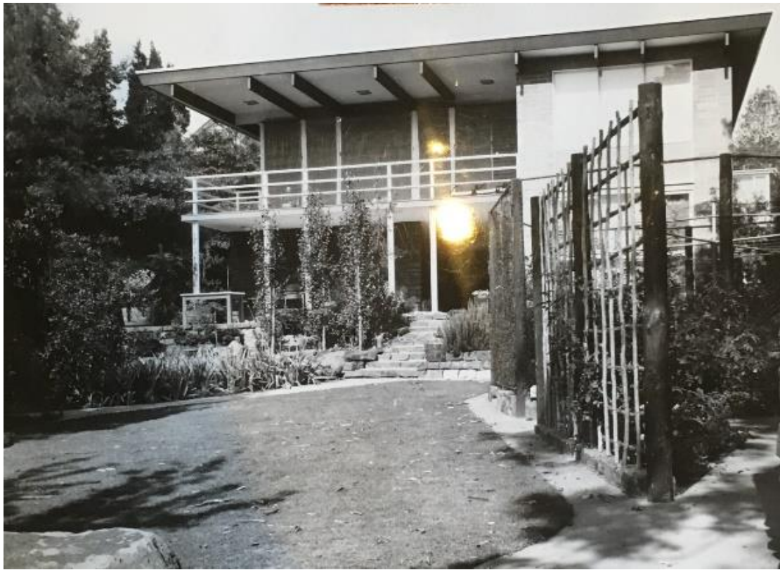
Figure 5: View of the rear of the house 2 years after construction of the garden. (Source: Mervyn Davis Papers 1950-1975, MS10706 State Library of Victoria)
