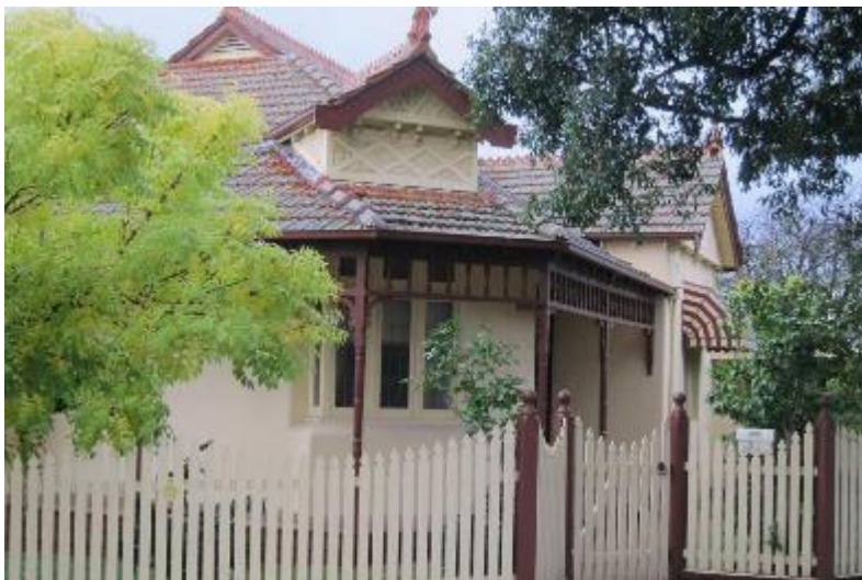
3 Manchester Street, a Federation house with corner orientation to Dixon Street. (Source: Context, 2017)
