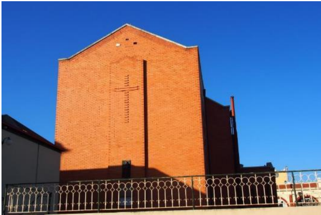
Figure 18. Rear, or northern elevation showing brick relief cross on the chancel exterior and the original fence around the plaza. (Source: Trethowan Architecture 2017)
