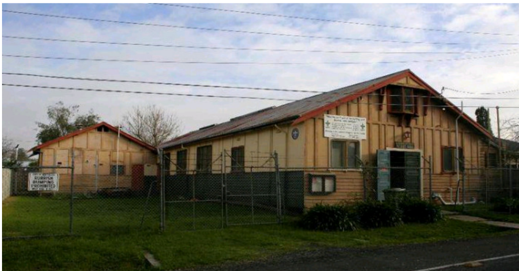
HO362 1st Alphington Boy Scout Hall no. 20 of 1931, Individually Significant place within Alphington East Precinct, City of Yarra (Source: VHD)
