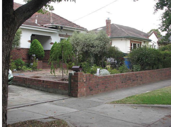
Streetscape: northern side of Maud Street, looking east
