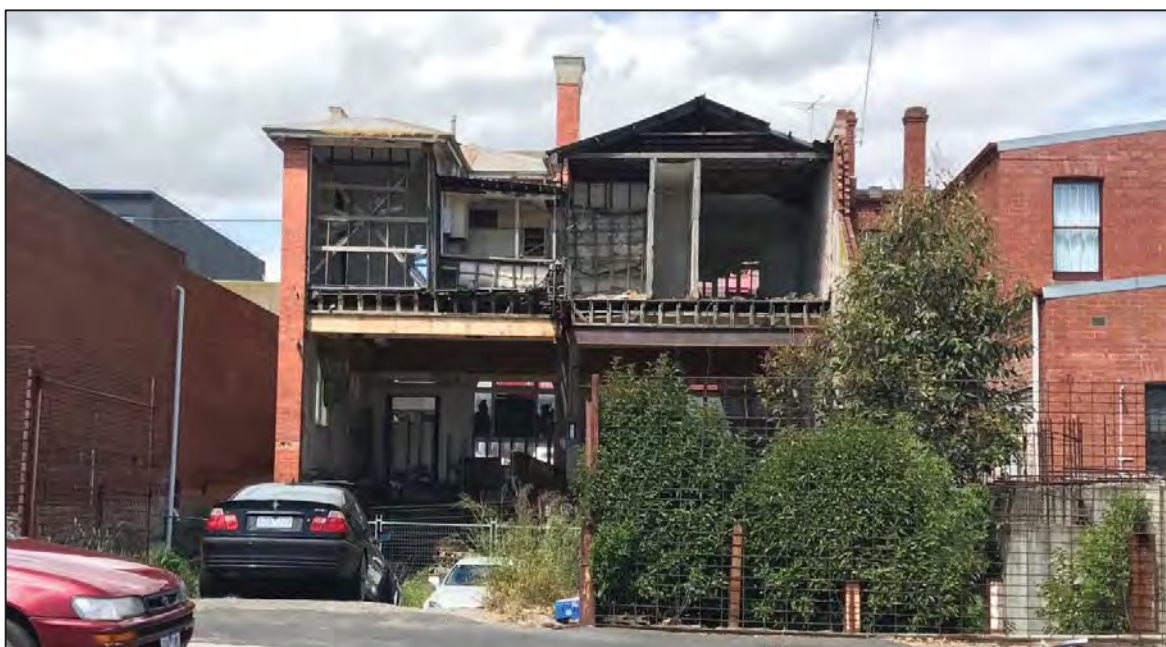
Above: Rear (west) of 851 Burke Road Camberwell
