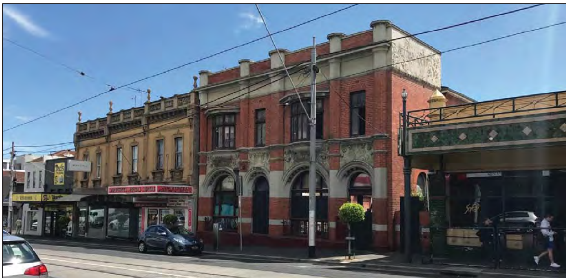
Above: the front façade of 851 Burke Road Camberwell (centre)
