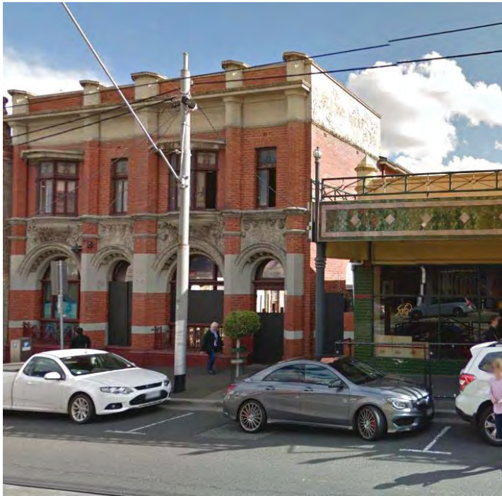
Above: The existing extent of visibility of the northern wall of the former State Savings Bank
