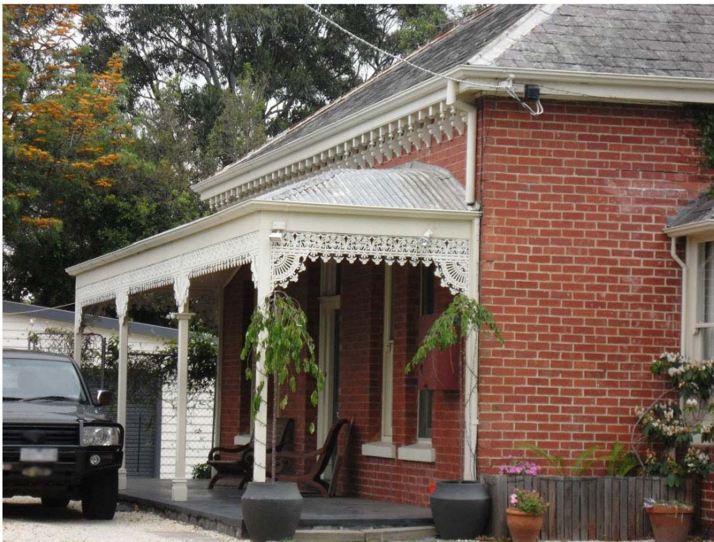
Figure 2. Detail of the original front façade (south elevation) with the decorative eaves brackets and reconstructed verandah. (Context, 2015)
