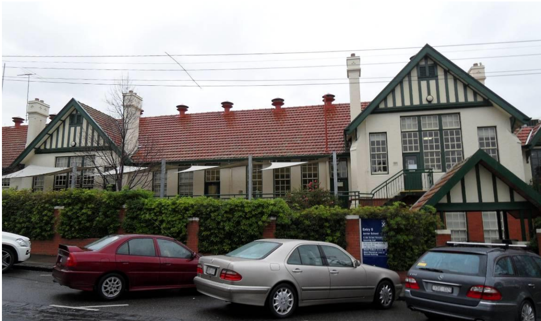
Figure 21. The original Preparatory School, north elevation, 2013.
