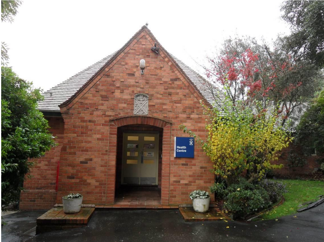
Figure 27. Front entrance of the Health Centre, 2013.
