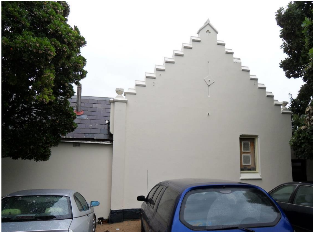
Figure 18. The Laundry, formerly part of a rear wing of 'Glen House' of 1874-75, 2013.
