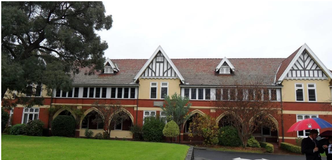
Figure 25. McMeckan House, north-west elevation, 2013.
