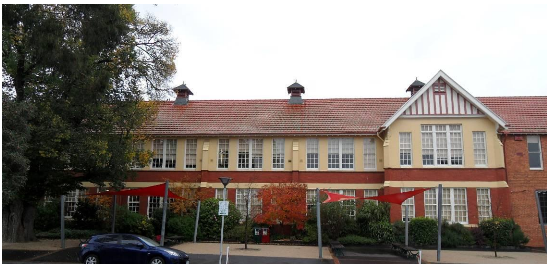
Figure 22. Main Quadrangle building, north elevation, 2013. Note the apricot brick section, right.
