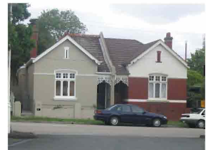
Precinct 2 - Burwood Road and housing
