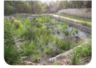
Image 1 Hambledon Street raingarden treating stormwater before it enters the Yarra River
