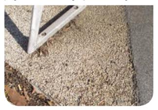
Permeable surfaces enable water to flow into the soil and eventually the groundwater
