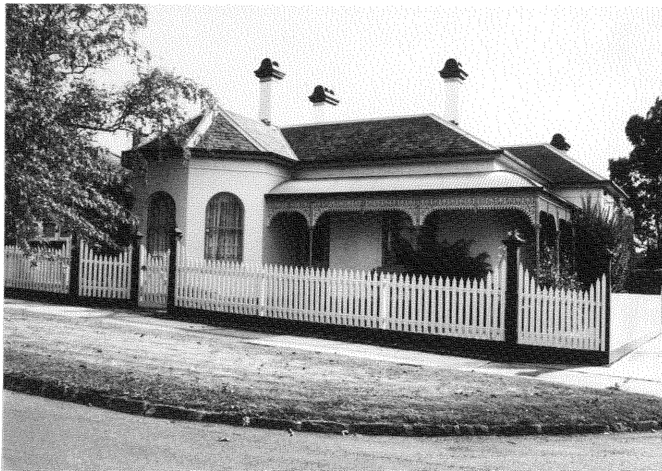
15 Smith Road (c1890) the typical Italianate villa, in this case finished in stucco and appointed with a cast-iron convex-roof verandah which returns down the side. The picket fence (new) is typical of many in the city's past where unlike the inner suburbs of Melbourne, there were few iron fences.
