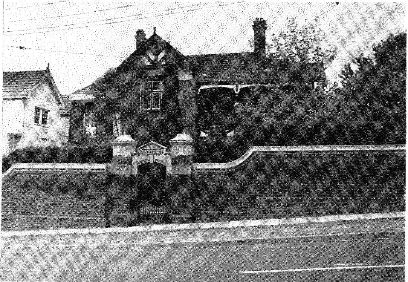
199 Whitehorse Road (1892) - half-timbering and oriels of medieval precedents: one of the prototypes of the Edwardian villas so numerous in Camberwell
