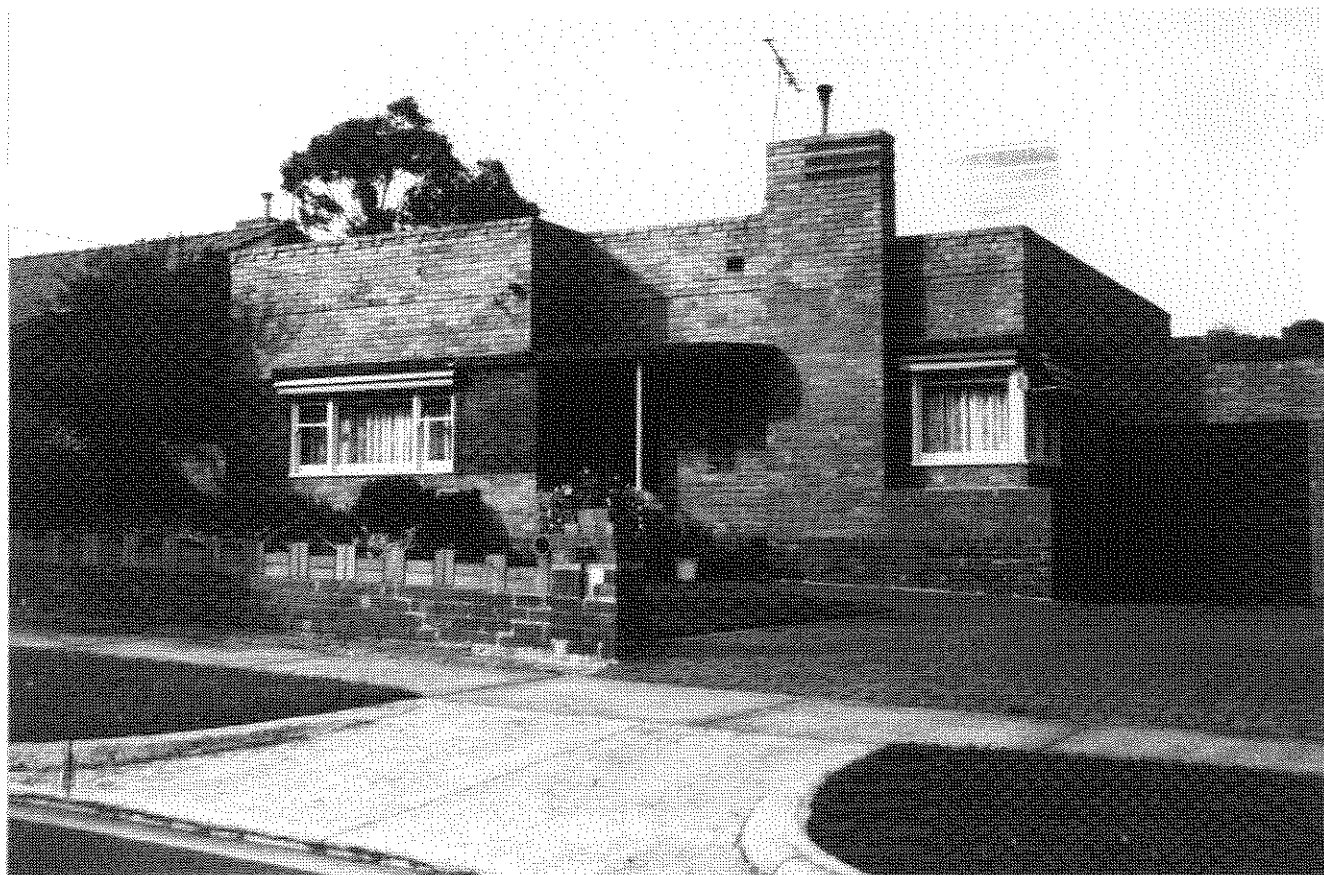
European Modern style house by the architects Seabrook & Fildes at 27 Hilltop Avenue: flat roof, banded brickwork and geometric forms overlapped for that cubist look.
