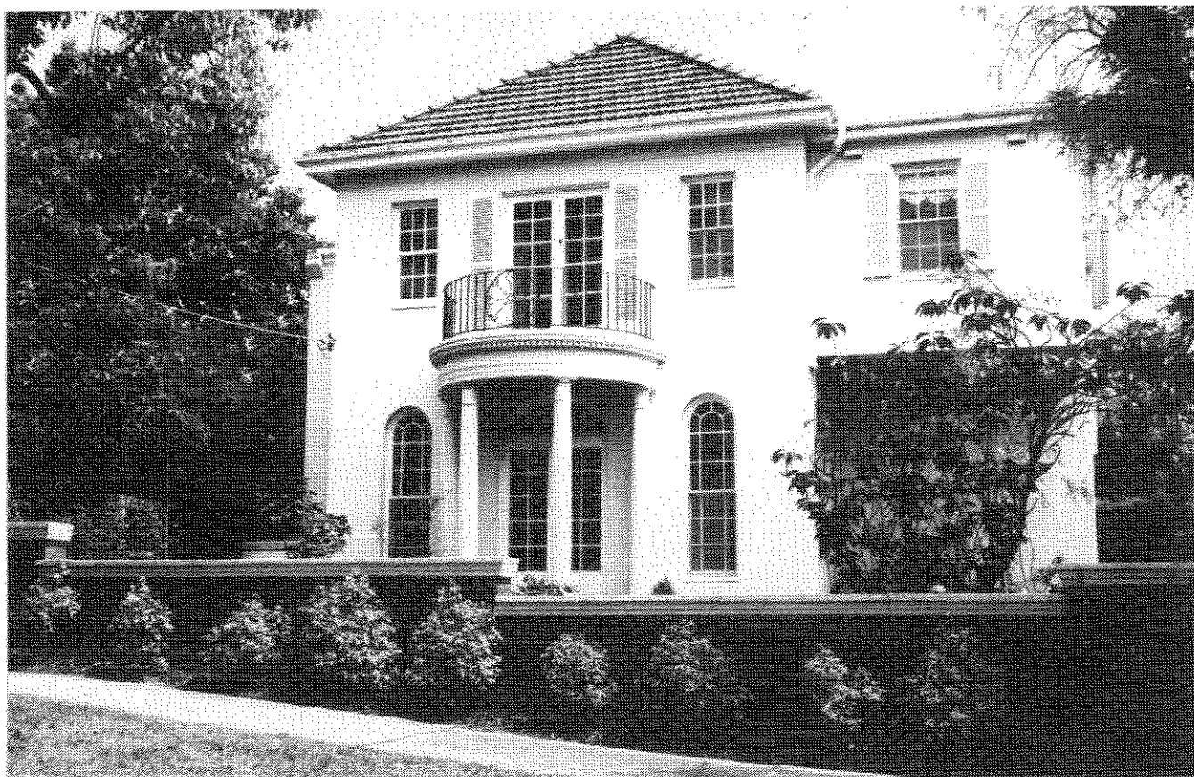
Fully developed Camberwell Neo-Georgian or Georgian revival, the symmetry, multi-paned glazing, classical entry porch and shutters (Crest Avenue, refer precinct 18)
