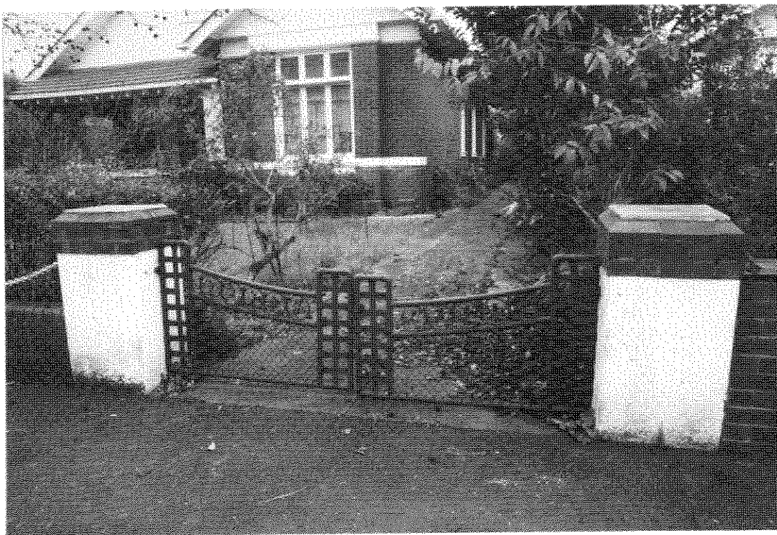
Detail of the fence and gate showing the typical drive with its twin concrete strips and the prevailing asphalt footpath paving which was used in late 19th and early 20th century estates.
