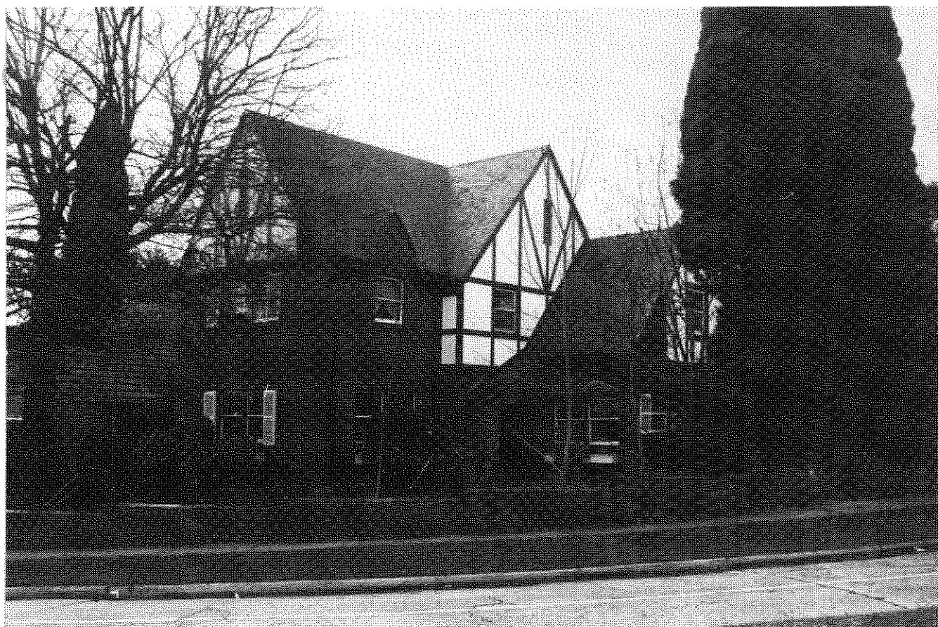
Old English style house of the late 1930s with clinker brick walls, shingle tile roof and half-timbered gables arranged in a picturesque way. The planting (cypress) and fence are as original fronting the concrete roads popular in the 1920-30s for estates (see precinct 18). The Old English or Tudor revival style houses were often noted in newspaper articles as very popular in Camberwell.
