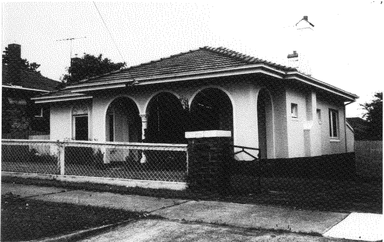
12 Catherine Street with its arcaded porch, stucco finish and hipped and tiled roof: all of the attributes of the Italian Villa style of the late 1920s early 1930s.
