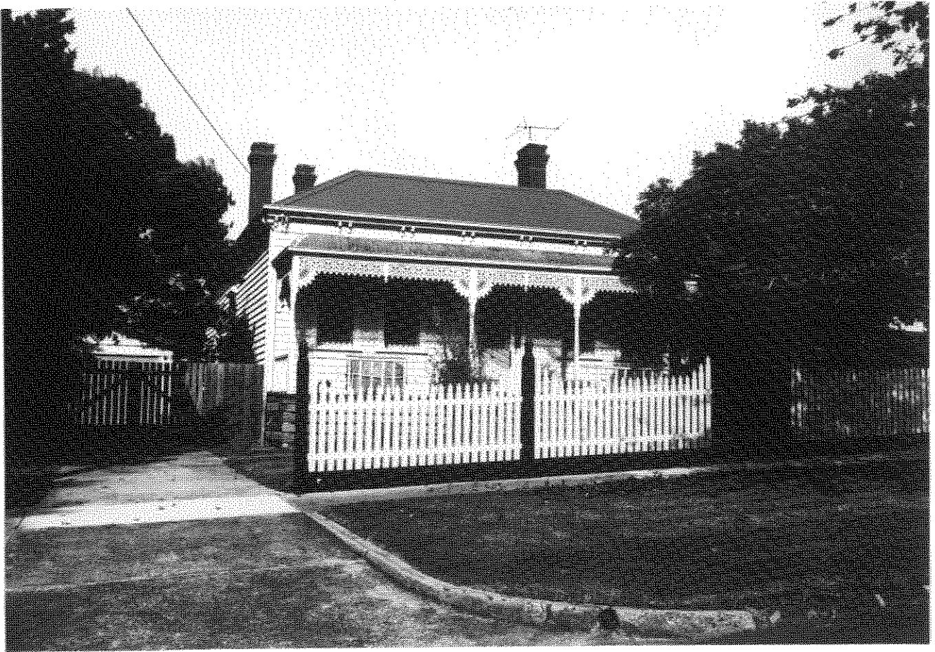
14 Smith Road (c1910) showing the lingering Italianate form but with the new Edwardian turned timber verandah posts bullnose verandah roof and an iron frieze pattern which was popular in that era. The new picket fence is also typical as are the brick chimney shafts with their corbelled brick cornices harking back to the Colonial type.
