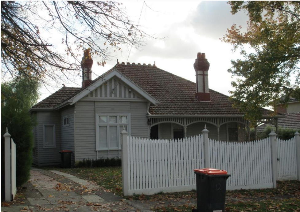
Figure 15 'Deansholme' at 12 The Avenue ('contributory'). A large Federation villa set on a generous block. The photo shows its condition prior to the addition of a new dormer window and garage in 2014.
