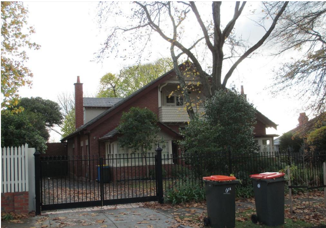
Figure 16 No.14 The Avenue ('significant'). A large bungalow house featuring a curved corner bay and large recessed upper balcony.
