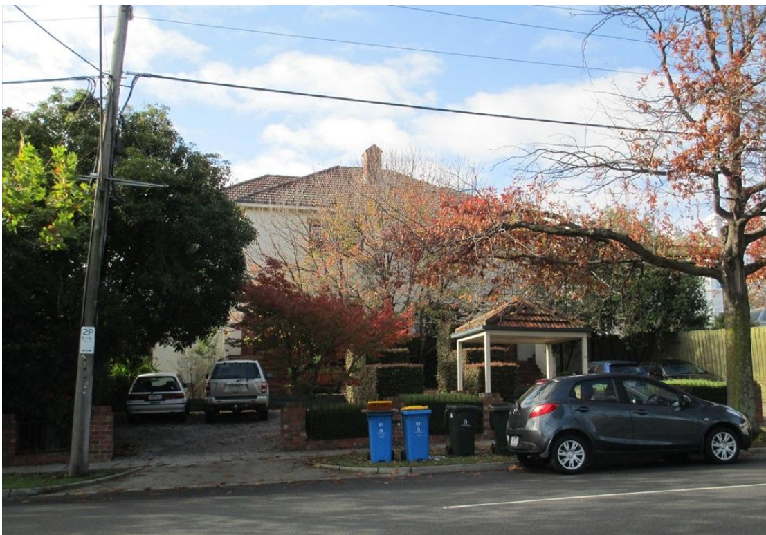
Figure 12 'Vista House', at 91 Union Road ('significant'). A rendered brick interwar duplex.
