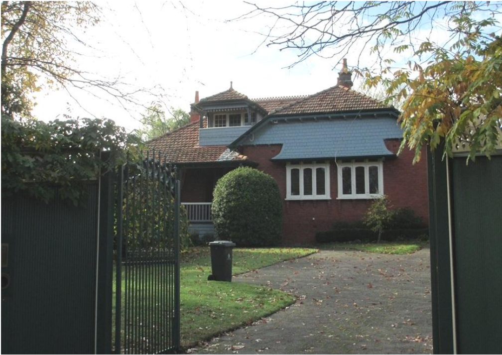
Figure 13 No. 83 Union Road ('significant'). A large red brick late Federation style residence with unusual details such as the jerkin headed gable and suspended curtain of shingles partly hooding a pair of fan lighted windows.
