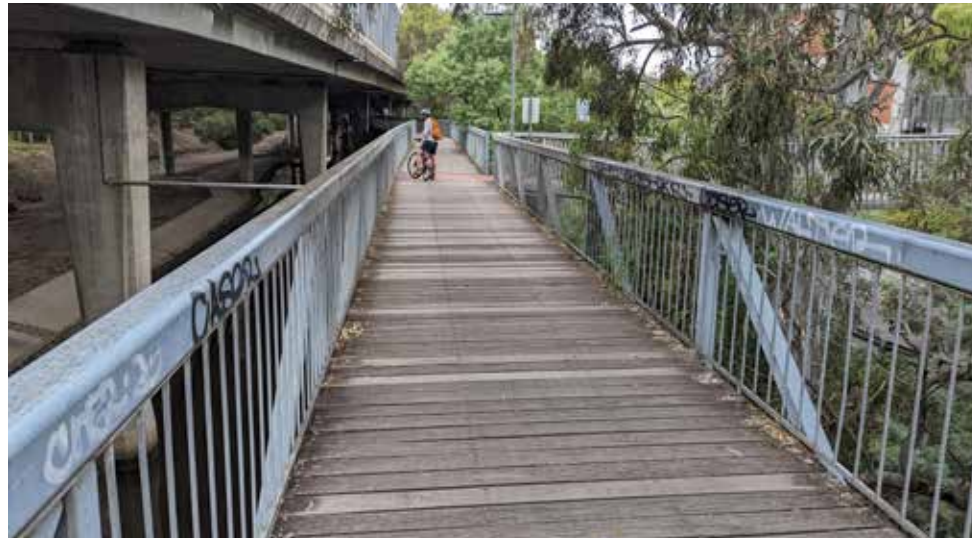
1 Underpass loose timber decking/narrow passage.
