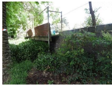
Figure 2.2 Bluestone retaining wall at south edge of former pétanque green, with cantilevered deck over part
