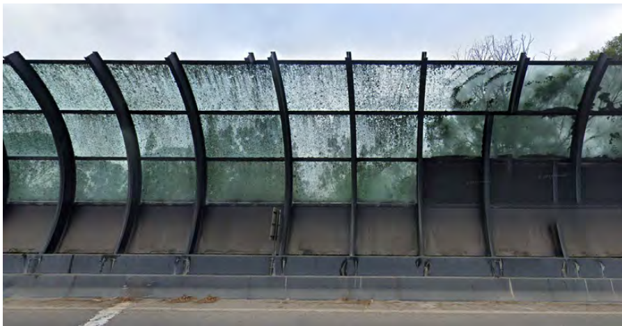
Condition of existing transparent noise walls near Jocelyn Avenue.
