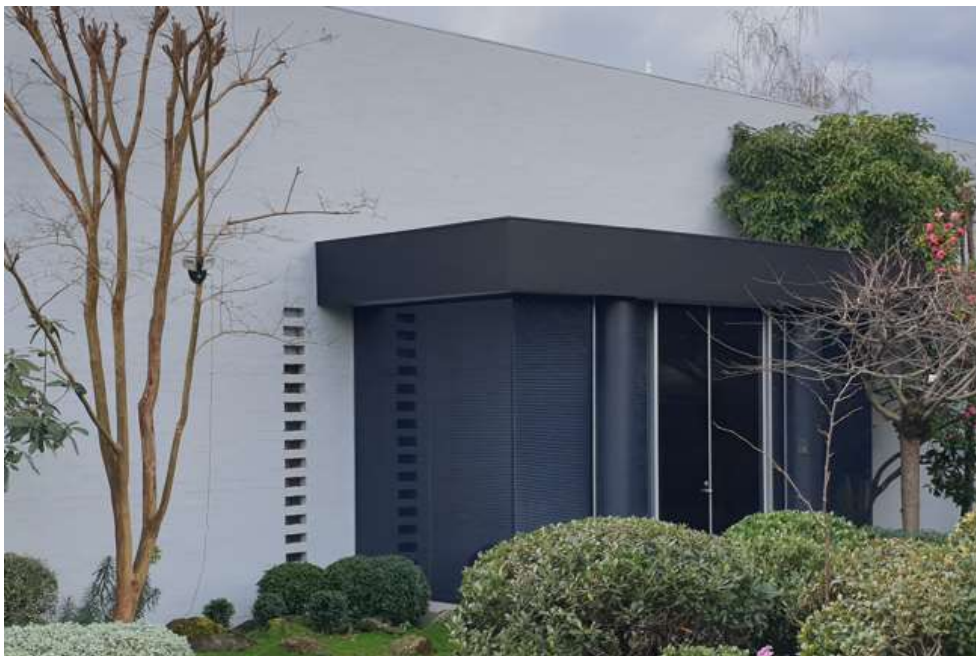
Figure 12 Street-facing south elevation of 57 Wattle Road, showing a stark, bagged wall of masonry with vertical a grill of hit-and-miss brickwork and fully glazed entry. Note: the hit and miss brickwork originally extended to the roof line. (Source: GML Heritage 2022)
