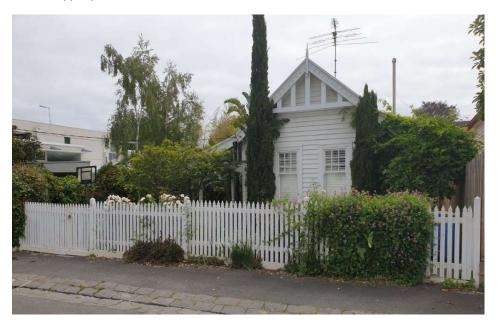
Figure 17 Timber house at 6 Wattle Grove, Hawthorn demonstrating characteristics of the Federation Queen Anne style with steeply pitched gable end with decorative barge boards and turned timber finial built c1907 (Source: GML Heritage 2021)
