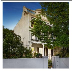
and relatively externally intact example of freestanding two-storey Victorian era terrace. The house displays characteristics generally typical of Victorian Italianate forms and detailing, including rendered brick walls, hipped slate roof behind a parapet, double-storey cast iron verandah set between wing walls, double-hung timber sash windows and a rendered brick chimney with Italianate cap. It forms a matching pair with 153 Power Street, which was built for the same owner in the same year.
