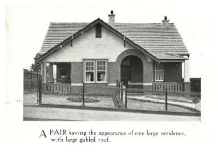
Figure 4 An example of a pair of residences designed to appear as a single Bungalow, this example from a Dunlop & Hunt catalogue. Dunlop & Hunt provided homebuyers with planning and construction services, as well as financing options. (Source: Dunlop & Hunt Home Builders Limited 1916:19)
