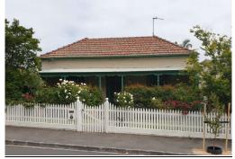
Figure 11 Rendered-brick Italianate villa at 32 Wattle Road, built c1889. The original slate or corrugated iron roof has been tiled and the verandah appears to have been altered (Source: GML Heritage 2021)
