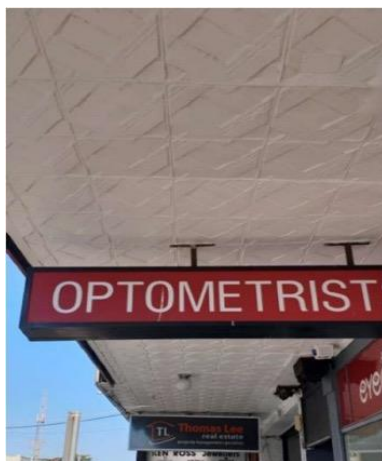
Figure 15. The soffit lining to the awning of 196-210 High Street (Source: Context 2019).
