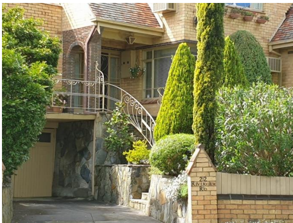
Figure 4 Detail of curved entry steps showing cladding to retaining walls and sub basements walls and mild steel balustrade. (Source: GML 2021)
