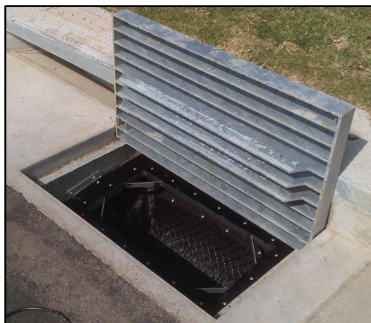
Figure 4.2: General configuration of the 200µm mesh SPEL StormSack
