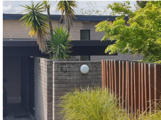
Figure 6 Concrete brick garden walls (integral to the original design) and timber fencing (recent) at the entry screening the front door from the street and creating an entry court. Note the integration of the carport roof over the top of the walls to give shelter to the front door. (Source: GML 2021)
