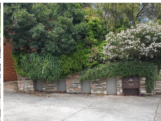
Figure 9 Stacked stone/retaining wall front fence, with integrated planter boxes and timber letterbox. (Source: GML 2021)
