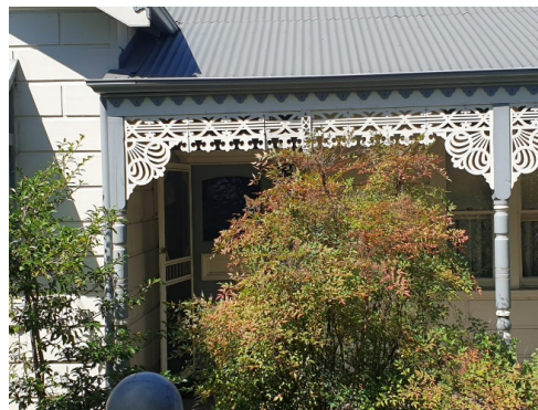
Figure 8. Detail of flat cast-iron frieze and brackets. Note the block treatment to the weatherboards to simulate ashlar stone. (Source: GML, February 2022)
