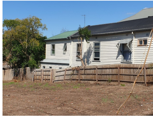
Figure 10. North (side) elevation of the house. Note the extant double-hung sash windows and window hood. (Source: GML, February 2022)
