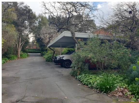
Figure 18 Contemporary photograph of carport, with view toward Wattle Road. Note the open pergola panel to the front of the carport has been filled in (Source: GML 2022)
