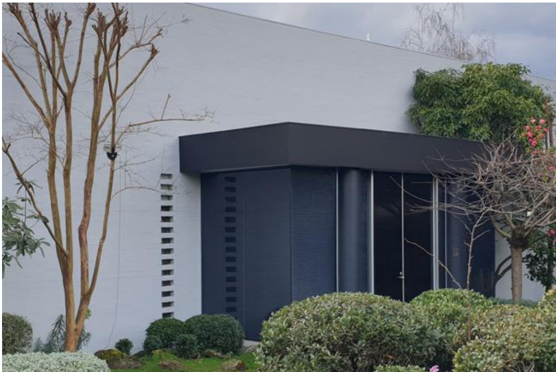
Figure 12 Street-facing south elevation of 57 Wattle Road, showing a stark, bagged wall of masonry with vertical a grill of hit-and-miss brickwork and fully glazed entry. (Source: GML Heritage 2022)
