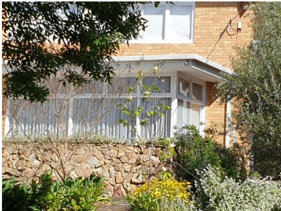
Figure 8 Detail of box bay window and uncoursed stone retaining wall to the front terrace. (Source: GML 2021)
