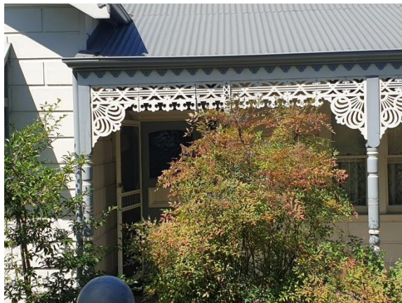
Figure 8. Detail of flat cast-iron frieze and brackets. Note the block treatment to the weatherboards to simulate ashlar stone. (Source: GML, February 2022)
