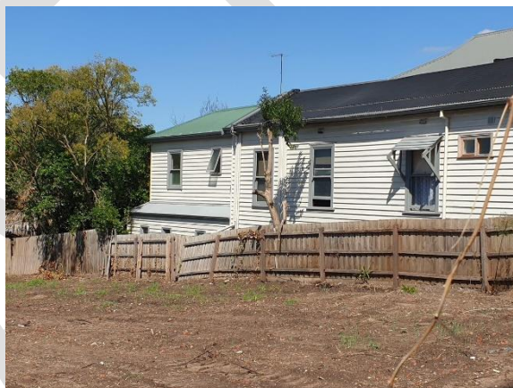
Figure 10. North (side) elevation of the house. Note the extant double-hung sash windows and window hood. (Source: GML, February 2022)
