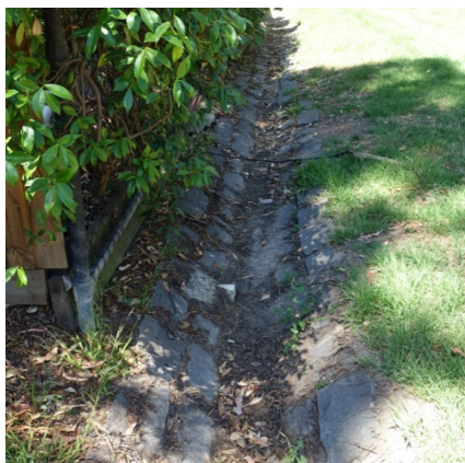
Figure 12. Deep bluestone pitched open channel to the rear of Roseberry Street, south side (Source: Landmark Heritage, 2022)
