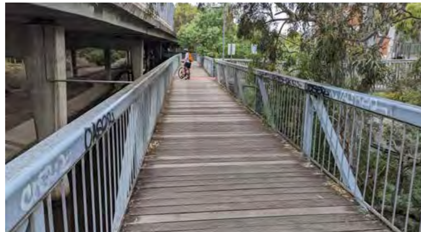
1 Underpass loose timber decking/narrow passage.
