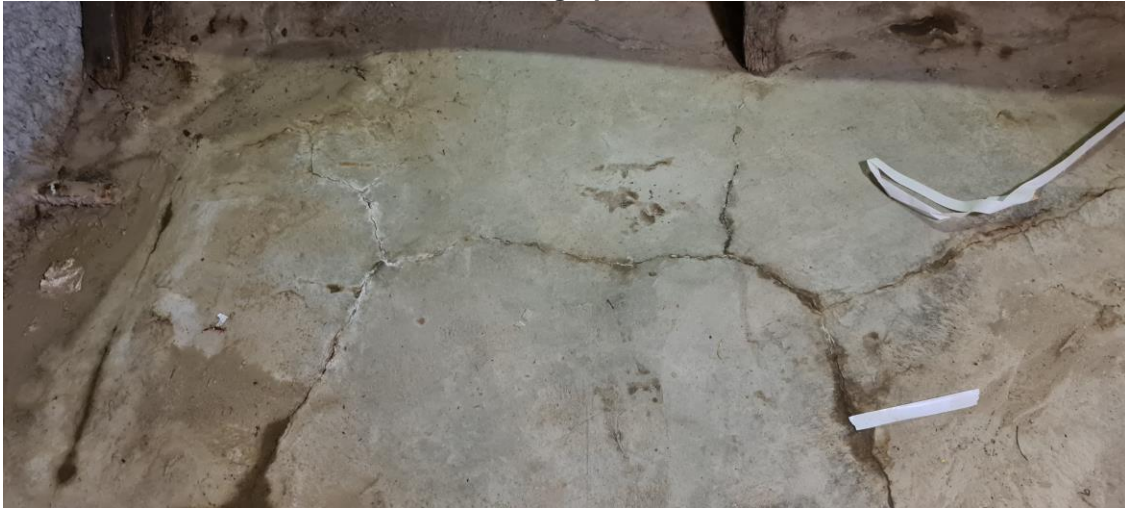
Photograph 9 – Surface cracks throughout the floor slab of the storeroom area
