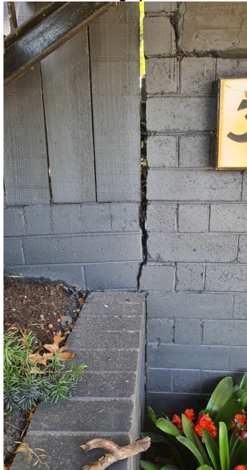
Photograph 17 – Brick wall separation between retaining wall and carport wall
