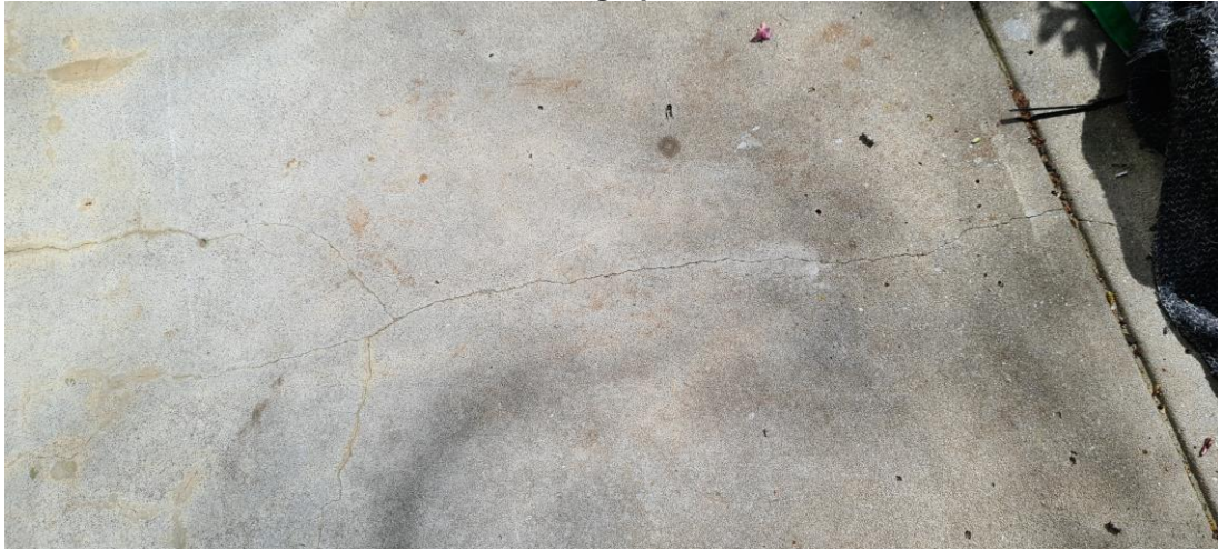
Photograph 27 – Hairline cracks on balcony floor slab
