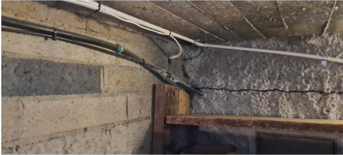
Photograph 15 – Horizontal crack along shotcrete wall
