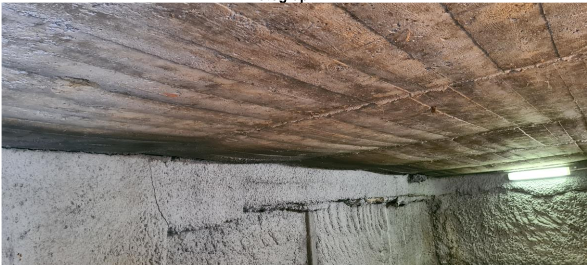
Photograph 12 – Upper floor concrete slab sagging
