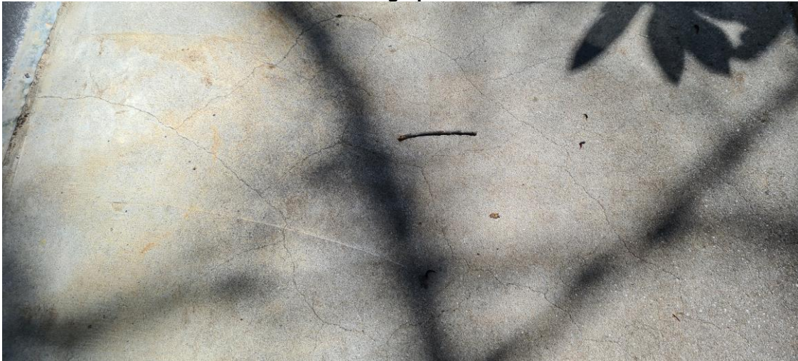
Photograph 28 – Hairline cracks on balcony floor slab
