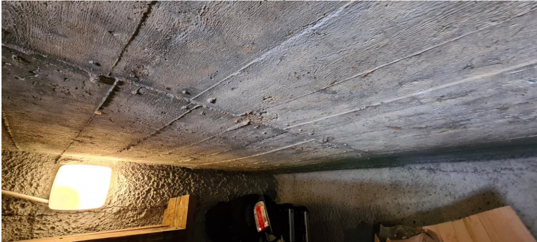
Photograph 13 – Upper floor concrete slab sagging
