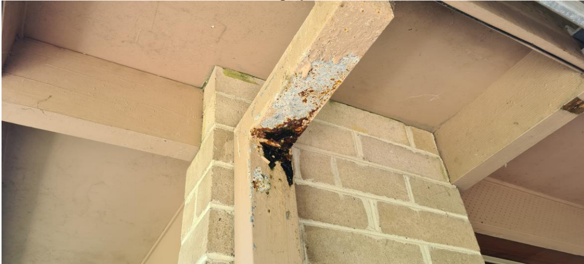
Photograph 25 – Corrosion of downpipe on east side of building
