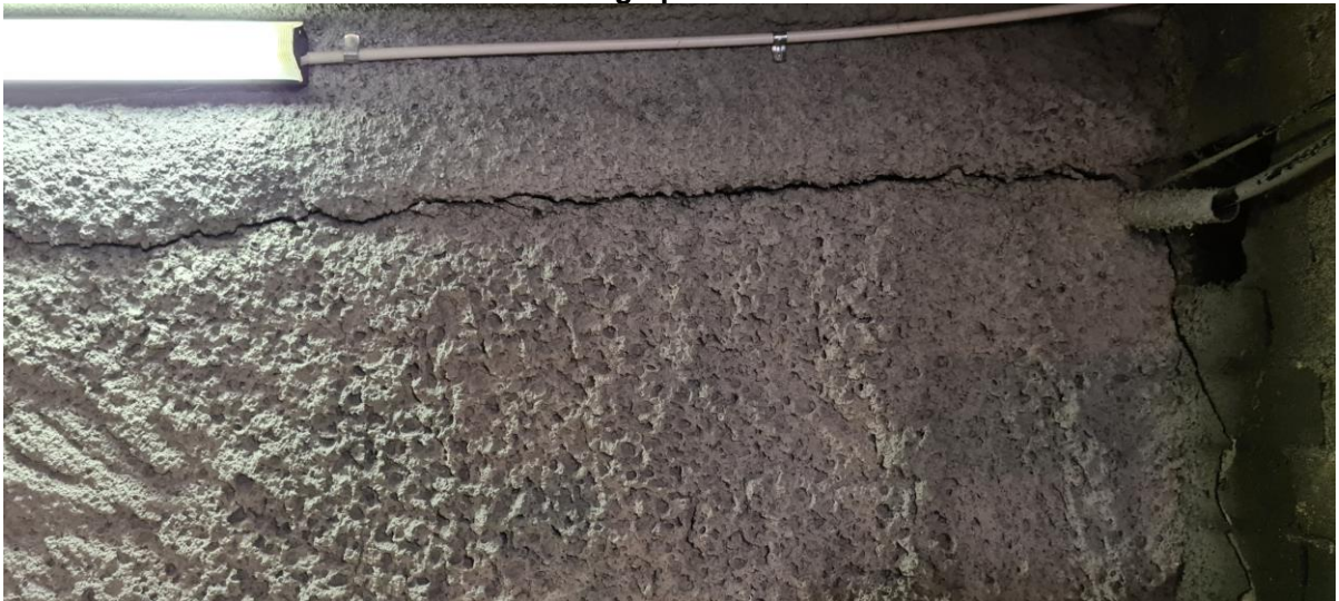
Photograph 4 – Crack along storeroom shotcrete wall assumed to be between capping beam and piles
