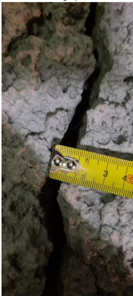
Photograph 6 – Vertical crack in the storeroom area shotcrete wall measured at 10mm
