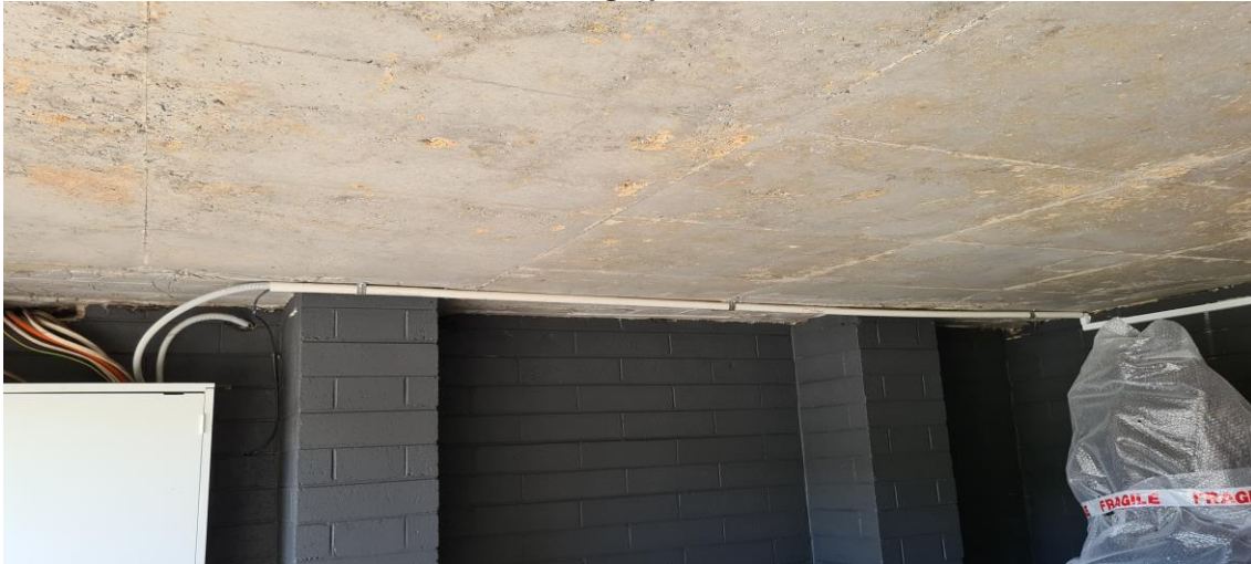
Photograph 21 – Concrete spalling and honeycombing present along the slab soffit in the carport area
