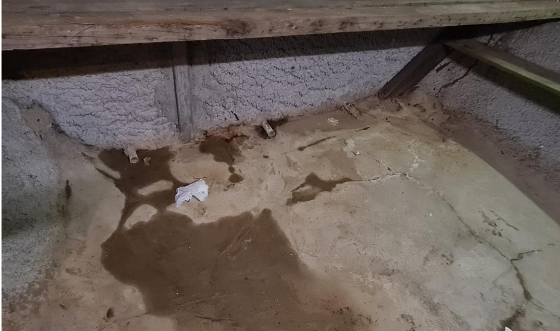
Photograph 1 – Pipes at the base of shotcrete wall for subsoil drainage
