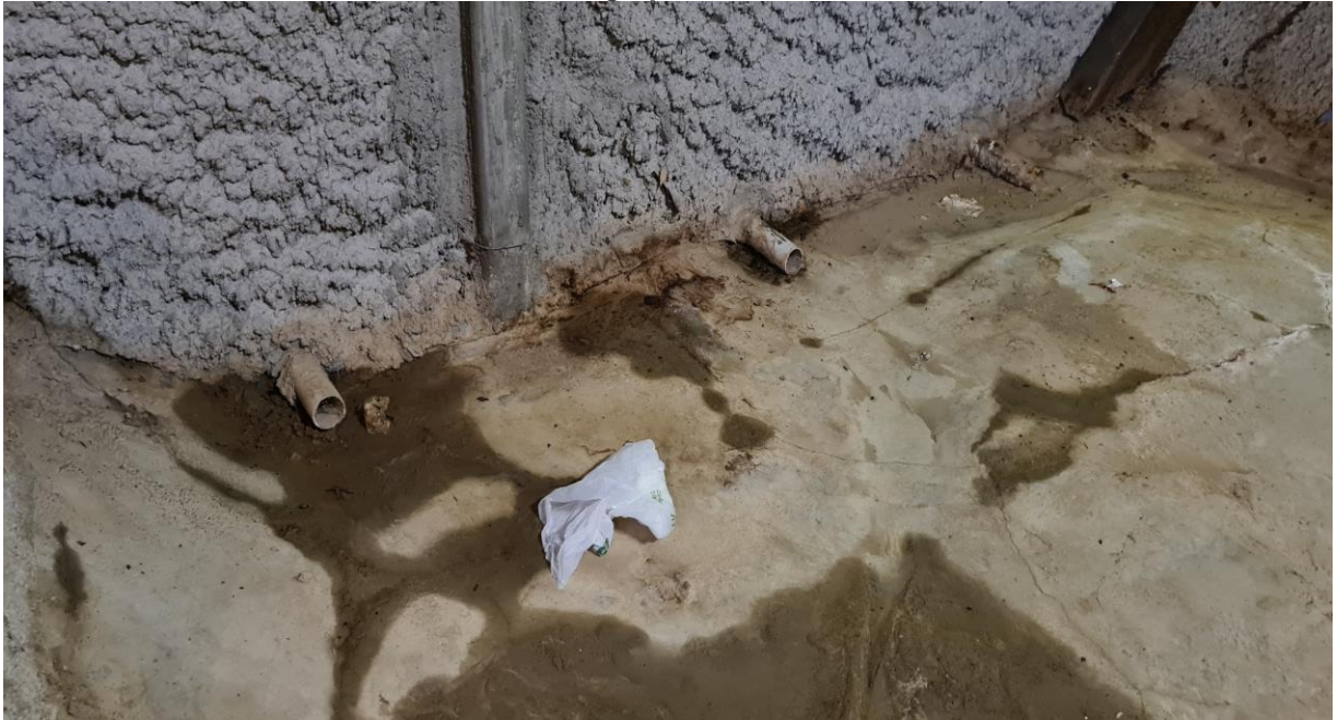
Photograph 3 – Excess moisture from shotcrete drain pipes
