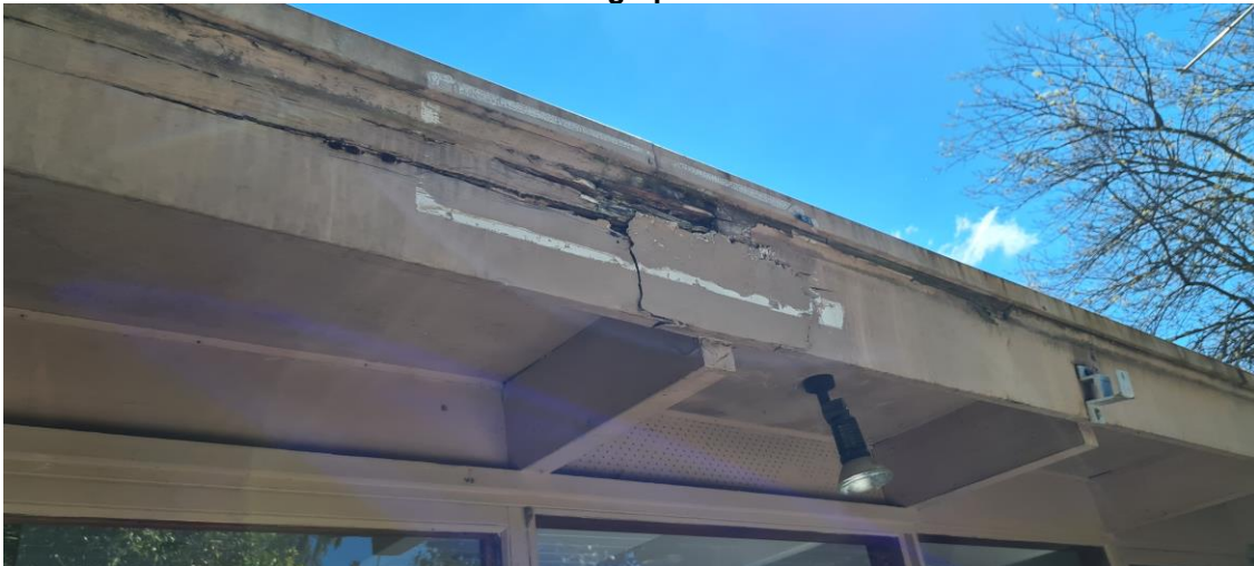
Photograph 26 – Timber fascia rot on east side of building
