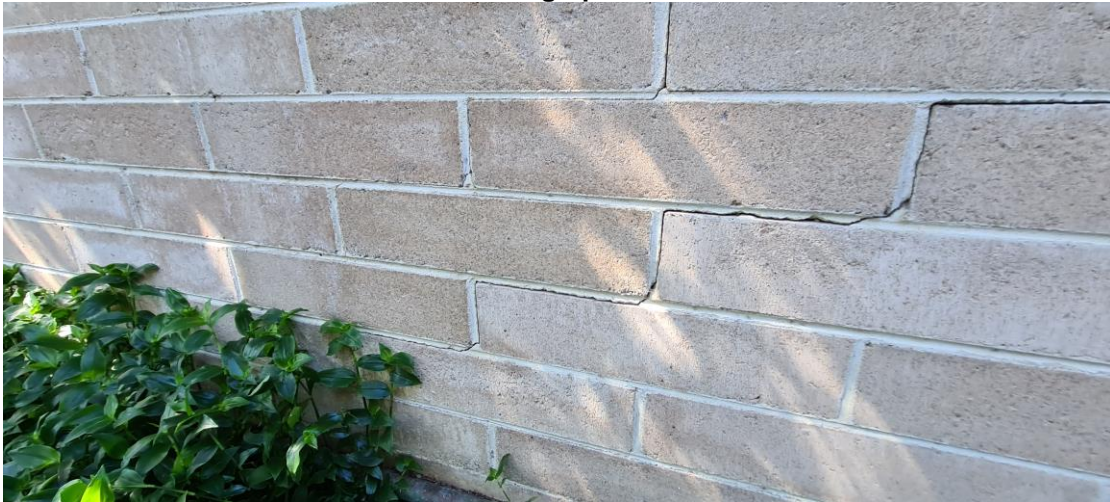
Photograph 24 – Continuation of stepped crack along west brick wall
