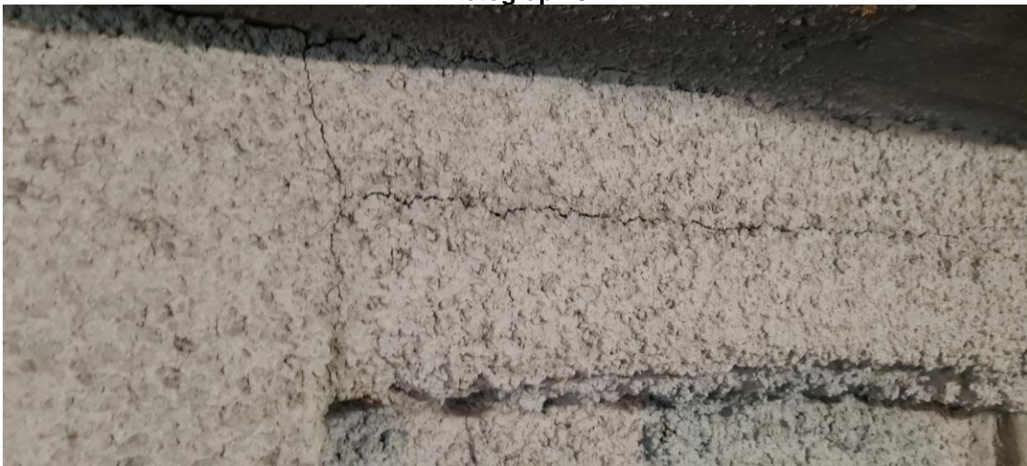
Photograph 8 – Cracks of up to 1mm appear throughout the surface of the shotcrete wall
