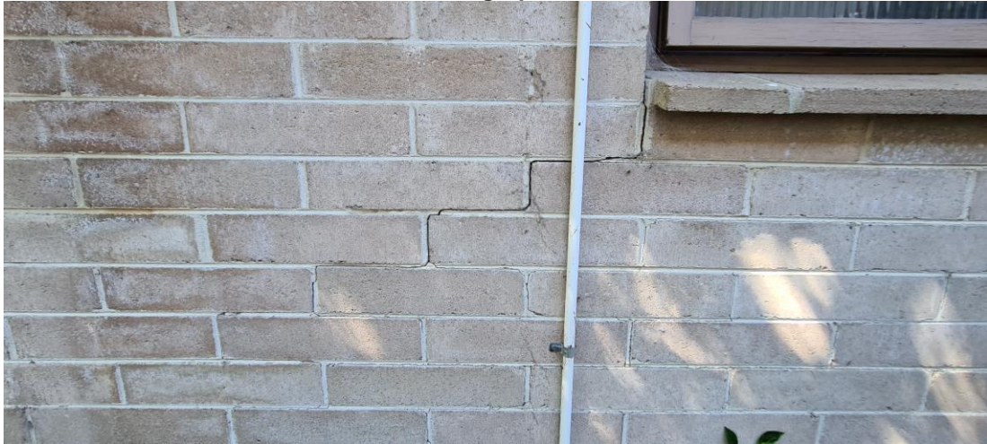
Photograph 23 – Stepped crack along west brick wall
