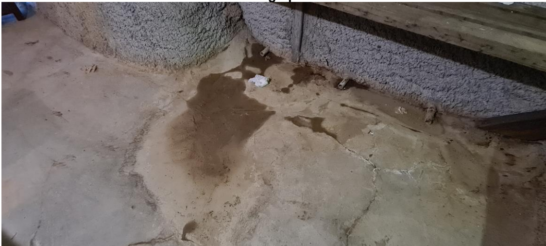
Photograph 2 – Subsoil drain pipes are draining into the storeroom area
