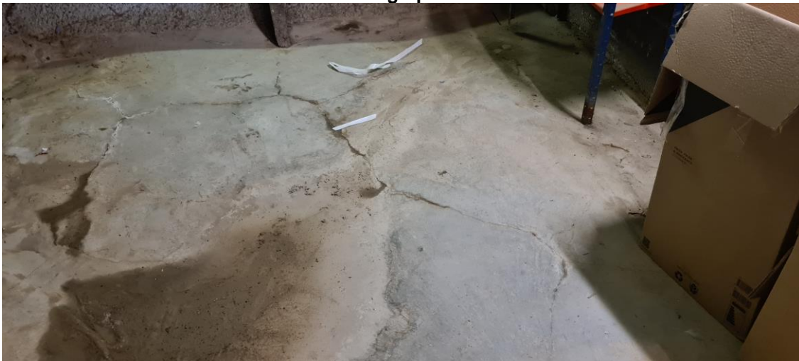
Photograph 10 – Water is ponding in areas where the floor slab has cracks
