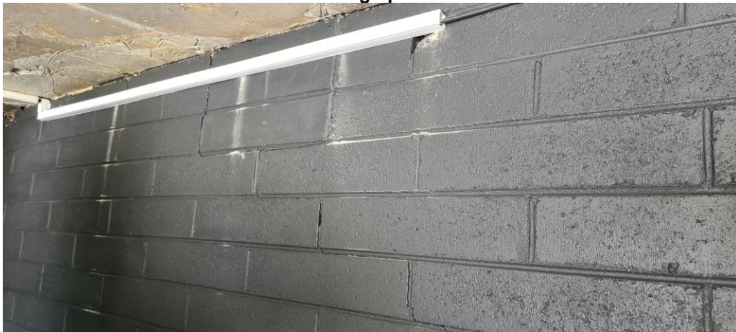
Photograph 18 – Stepped crack in brick wall between carport and storeroom
