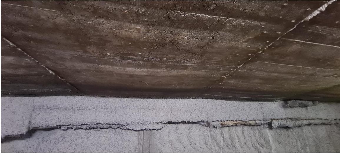
Photograph 11 – Upper floor concrete slab sagging
