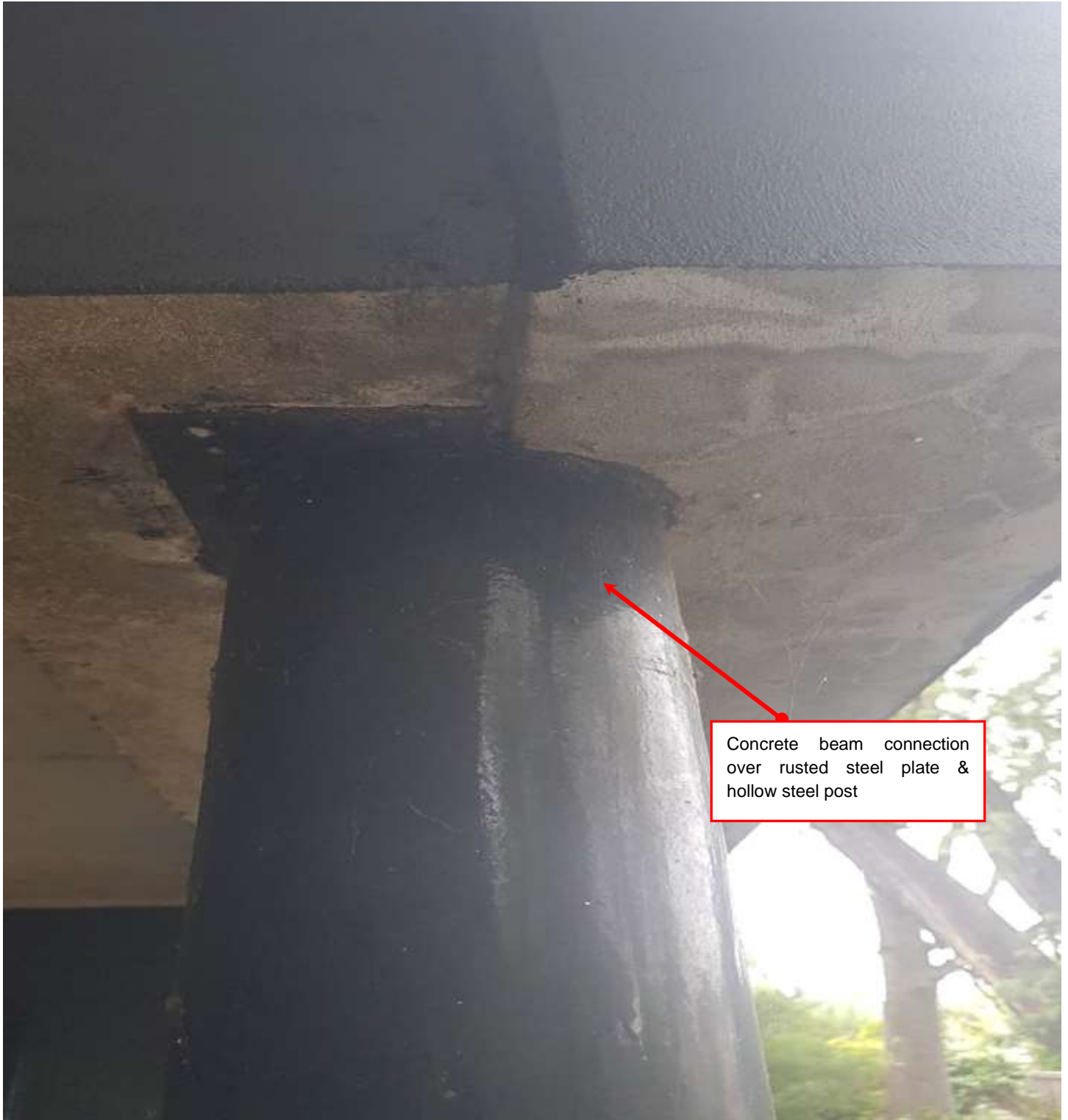
Photograph 5 – Concrete slab rusted support
