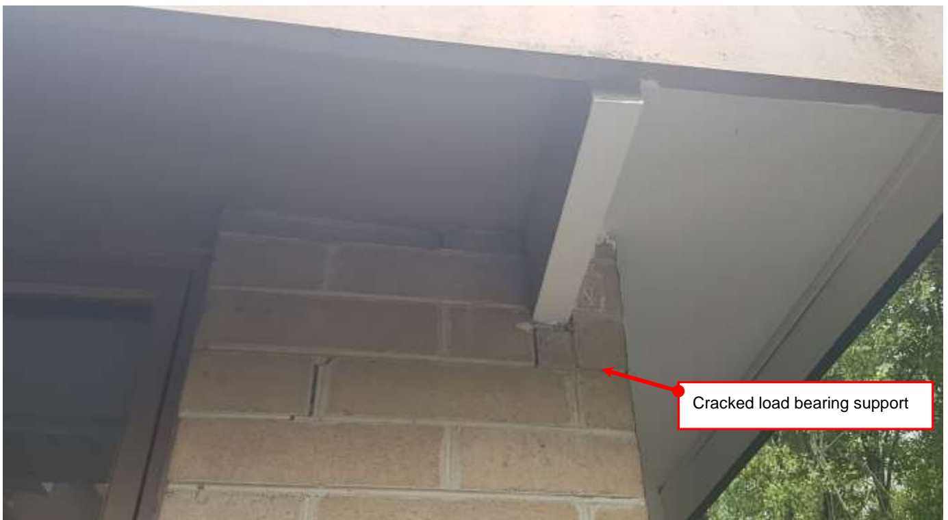
Photograph 11 – wall above basement
