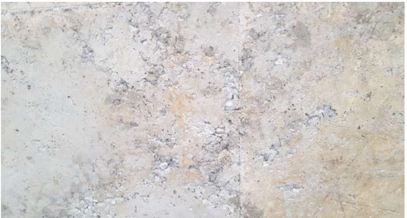
Photograph 10 – Poor quality concrete slab
