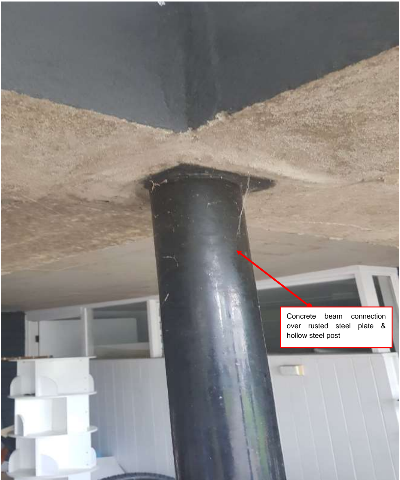
Photograph 6 – Concrete slab rusted support
