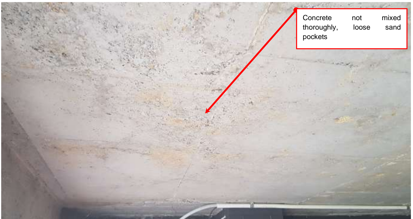
Photograph 8 – Poor quality concrete mix with loose sand pockets
