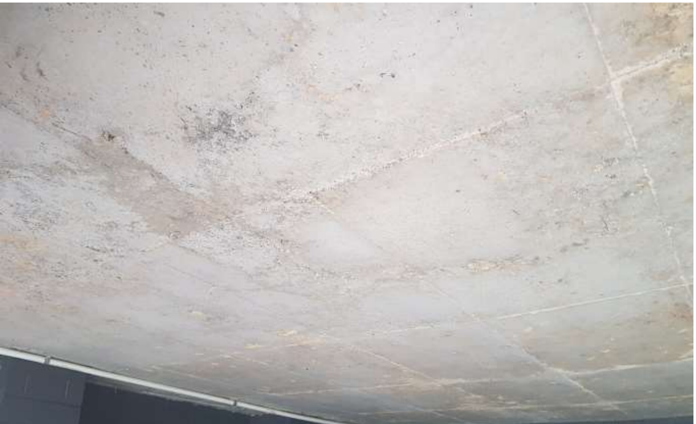
Photograph 9 – Poor quality concrete slab
