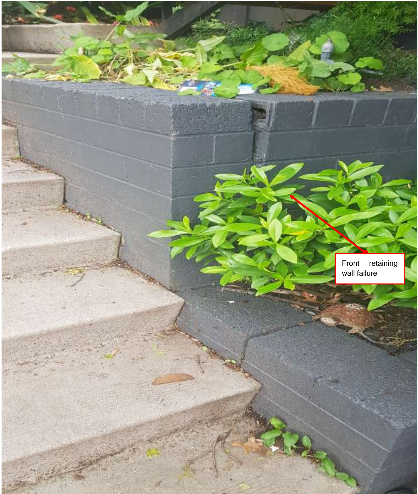
Photograph 3 – Cracked retaining wall
