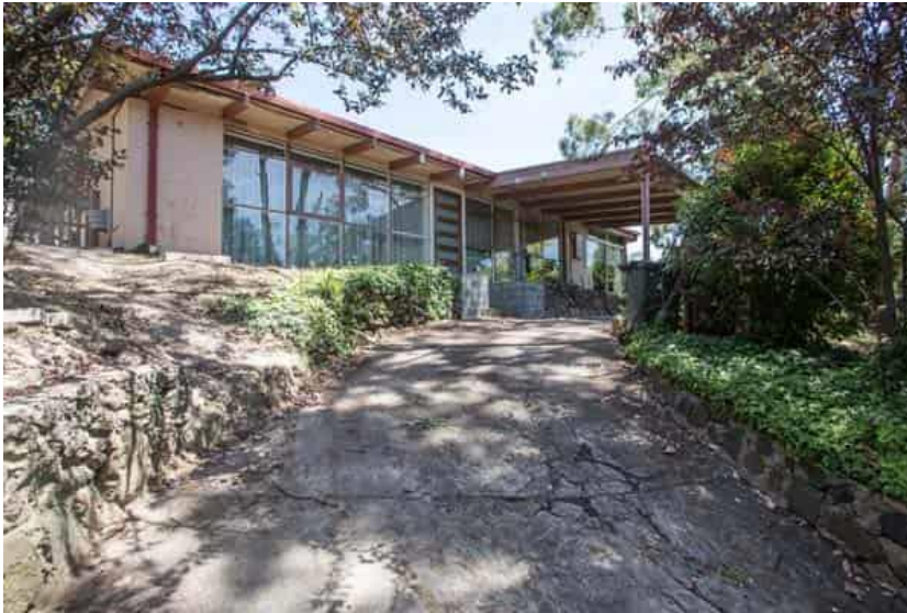
Figure 32 'Dome 12' One of the houses Knox designed for the Hillcrest Estate with non-load bearing internal stud walls, a Stramit ceiling and a malthoid and gravel roof (usually replaced). Photo: Tony Knox Source: AlistairKnox.org: https://alistairknox.org/buildings/55
