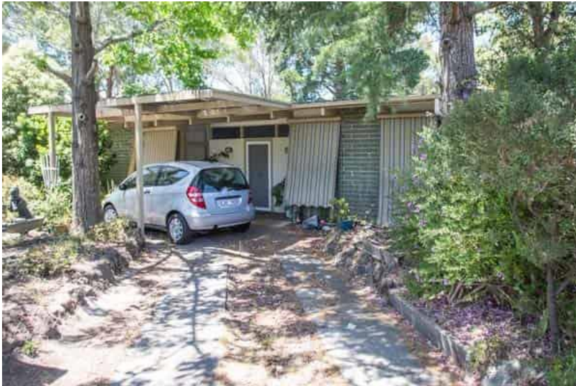
Figure 25 'Dome 32' One of the houses Knox designed for the Hillcrest Estate with non-load bearing internal stud walls, a Stramit ceiling and a malthoid and gravel roof (usually replaced). Photo: Tony Knox Source: AlistairKnox.org https://alistairknox.org/akimages/636
