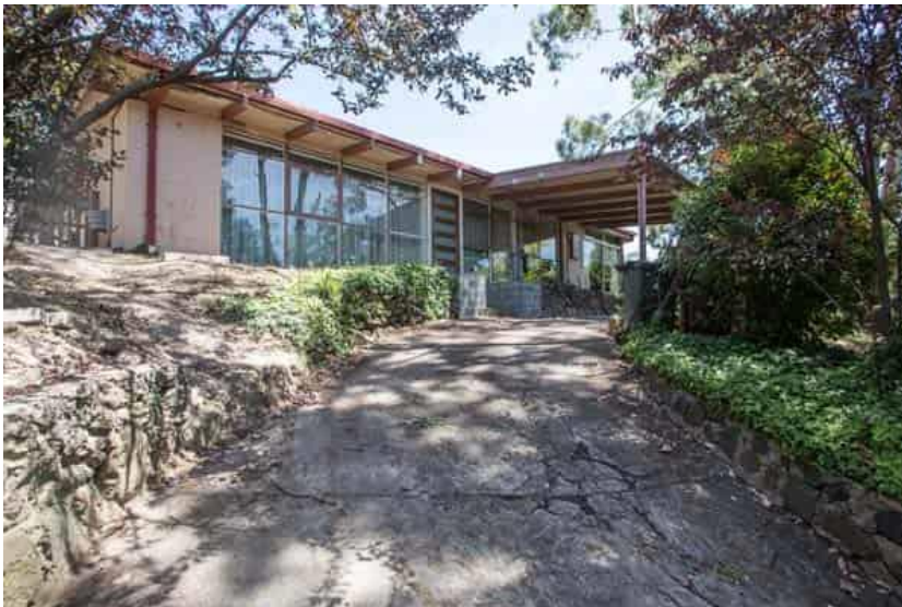
Figure 24 'Dome 12' One of the houses Knox designed for the Hillcrest Estate with non-load bearing internal stud walls, a Stramit ceiling and a malthoid and gravel roof (usually replaced). Photo: Tony Knox Source: AlistairKnox.org: https://alistairknox.org/buildings/55
