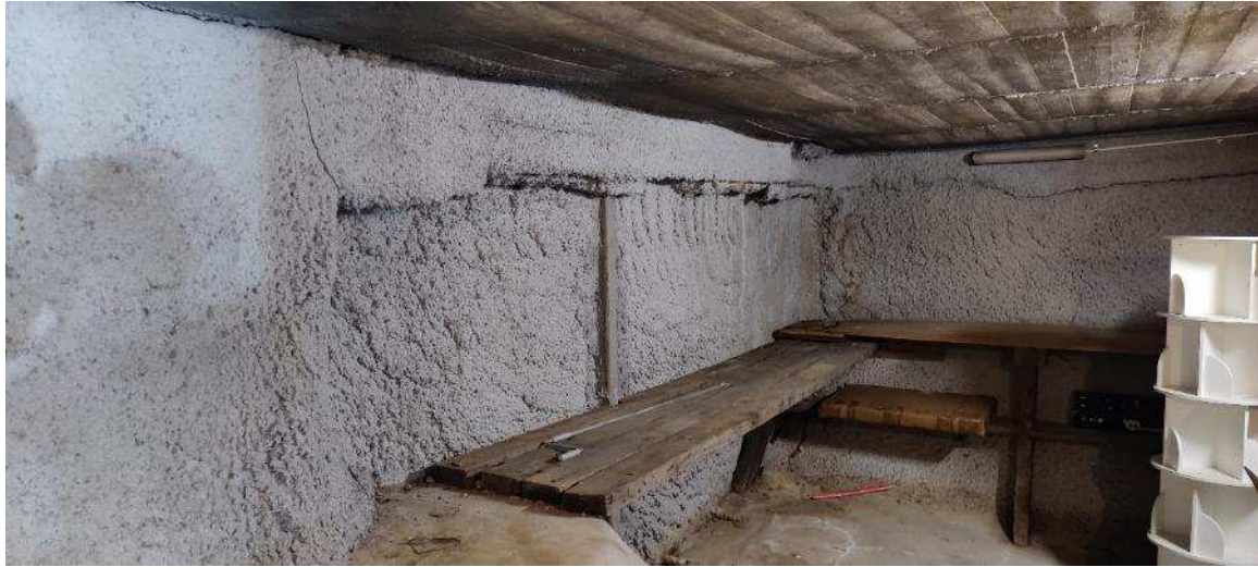
Figure 8: Storage area at rear of the undercroft. Note the shotcrete to the retaining walls. The concrete slab to the floor above is noticeably bowed in this image. Source: Trethowan Architecture, 2022.
