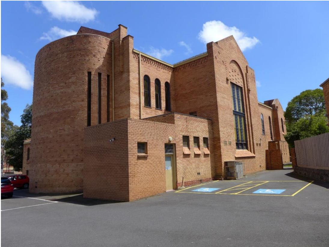
Figure 16. The church viewed from within the carpark at the rear of the site. Note the Romanesque massing, decorative brick work in the tympanum over the transept window, and a corbel table under the roofline. The square toilet block in the foreground is a later addition. (Source: Trethowan Architecture 2018)
