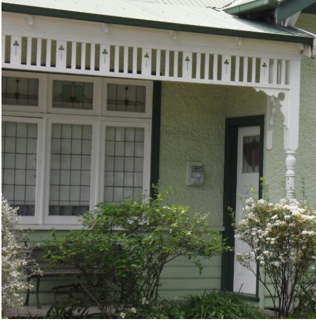
Figure 3. Details around the front entry of 9 Donald Street: weatherboard and roughcast cladding, verandah fretwork, leadlight windows and high-waisted door. (Source: Context 2019)
