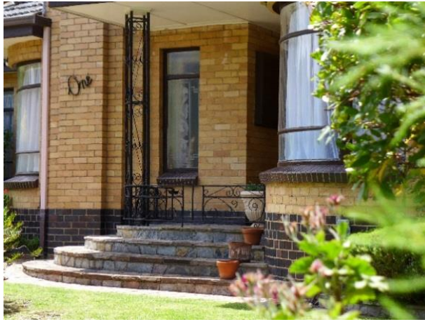
Figure 6. The entry porch, with floral motif frosted glass in the adjacent window and ironwork pier and balustrade. (Source: Trethowan Architecture 2018)
