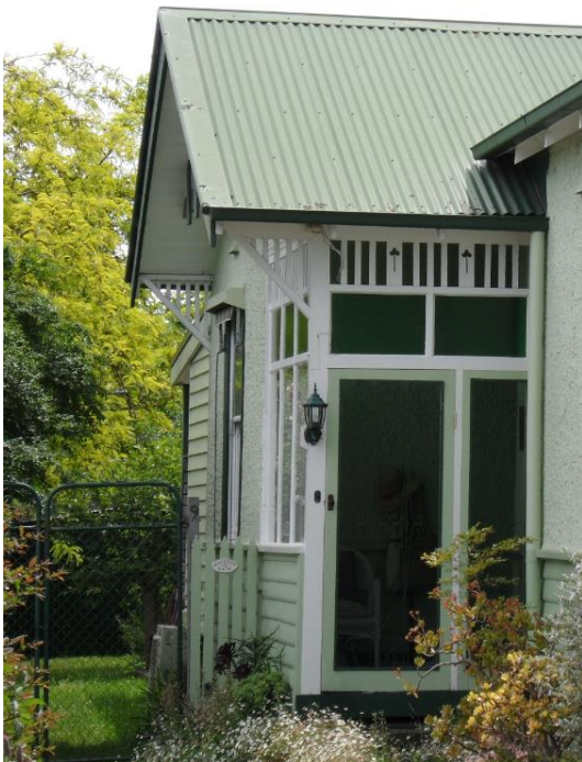
Figure 4. Side entry porch with timber fretwork, ladder-back brackets and reen glass. (Source: Context 2019)
