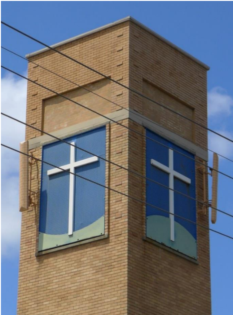
Figure 17. Detail of the top of the tower, showing screen over the belfry and sympathetic brick extension on top. The original frame and decorative features remain, and the screen appears to be detachable. Mobile telecommunications equipment has been attached to the tower. (Source: Trethowan Architecture 2018) Comparative Analysis
