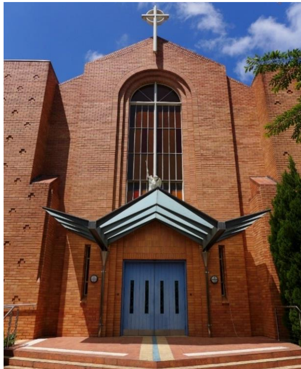
Figure 13. Front view of the central façade, showing original door, with statue above, dominant brick massing, large central arched window within simplified archivolt. The steel and glass canopy is a recent addition. (Source: Trethowan Architecture 2018)
