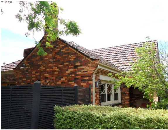
Figure 7. Vergeless gable end and corbelled glazed brick eave detail at 6 Dunlop Street, Ashburton. (Source: Context 2019).
