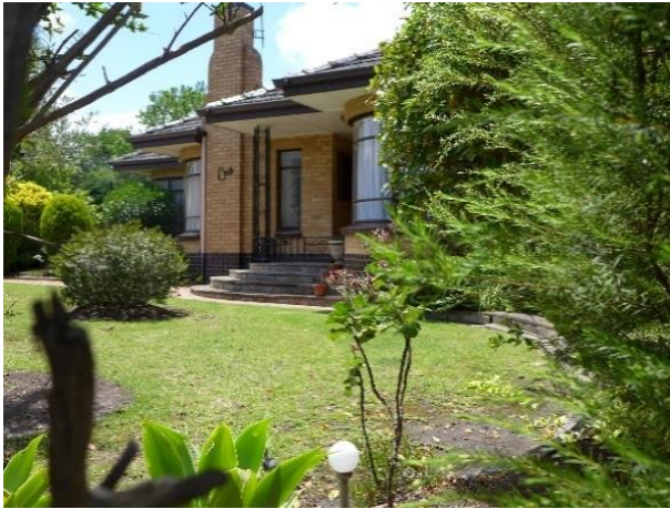
Figure 5. View of the façade of the house showing waterfall chimney and hipped roof. (Source: Trethowan Architecture 2018)
