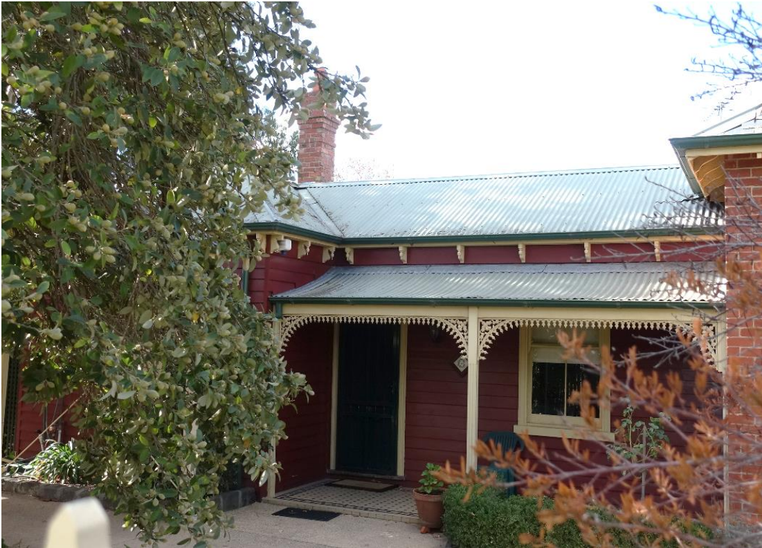
Figure 13. West (original front) façade of the c1885 house. Note the asymmetrical façade, concave verandah, and two-over-two sash window. (Source: Context, 2019)
