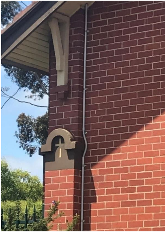
Figure 9. Detail of concrete arch mouldings with cross on pier and bracket under eave. (Source: Trethowan Architecture 2018)
