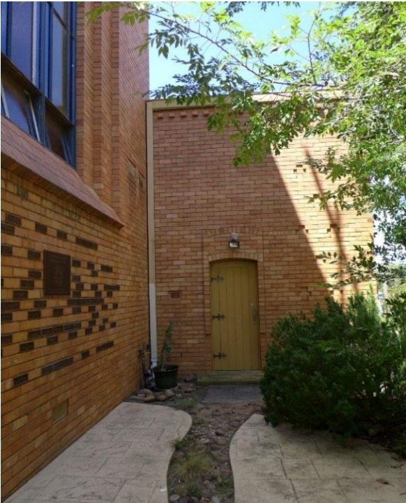
Figure 12. Detail of Sacristy entry showing brick detail over door suggesting a dripstone moulding, embossed brick crosses, and brick dentil pattern at top of the wall. Memorial Garden plaques on the left. (Source: Trethowan Architecture 2018)
