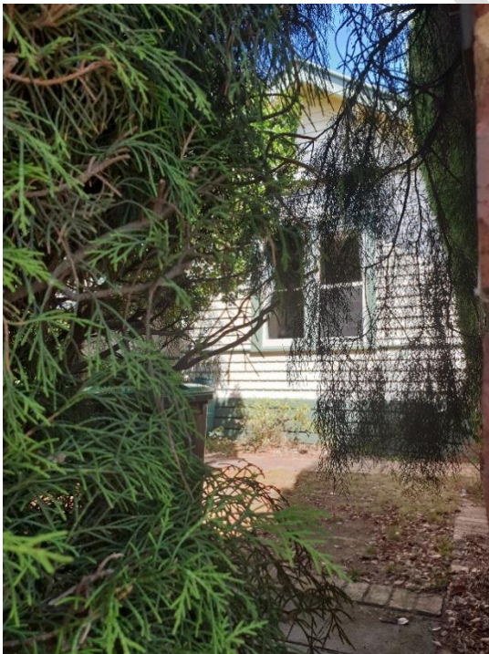
Figure 12. View of the north-facing projecting bay at 41 Austin Street, Balwyn, showing paired double-hung sash windows set in a decorative architrave. Note the timber mould at sill height, below which the weatherboards are notched. (Source: GML February 2022)
