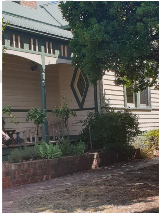
Figure 13. View of the diamond-shaped leadlight window under the verandah at its western end. Note the turned timber verandah posts and decorative fretwork. (Source: GML February 2022)
