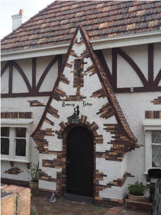
Figure 7. Detailing of brickwork, arrow slit and tiles around entrance gable (Source: Trethowan Architecture, 2018).
