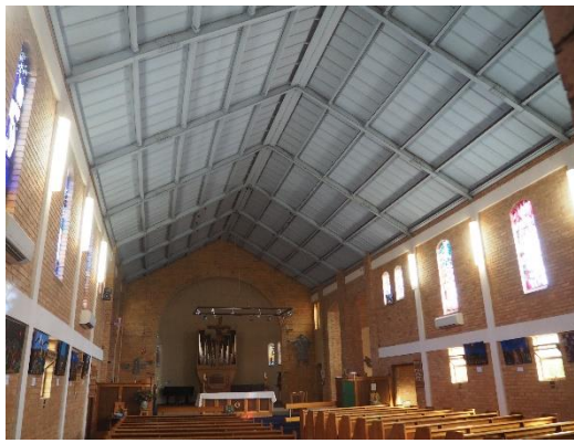
Figure 11. Interior view of the Church. Note the cream brick walls and expressed portal frame structure. (Source: Trethowan Architecture, 2018)
