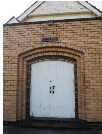
Figure 12. The main entry to the former timber chapel with its stepped arched entrance with brown brick surrounds and base. (Source: Trethowan Architecture 2018)
