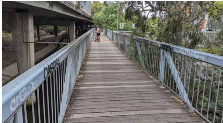
1 Underpass loose timber decking/narrow passage.
