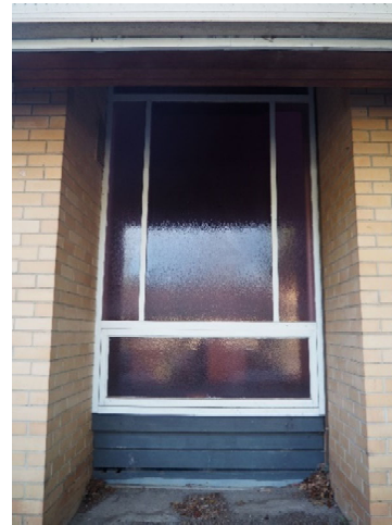
Figure 10. Modular stained-glass windows as found between each of the side elevation buttress forms. (Source: Trethowan Architecture, 2018)
