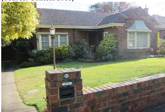
Figure 17. Early post-war Old English house at 62 Brandon Street (1948). Note the clinker brick, canted bay window with bell-cast eaves, low gable slope and corner window. (Source: Context 2018)
