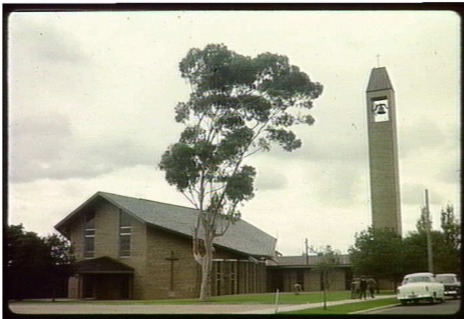
Figure 22. View of North Balwyn Uniting Church from Duggan Street in 1964-65, photograph by Peter Wille. Note the unusual roof form created by the octagonal plan and the very tall, detached bell tower. (Source: State Library of Victoria)
