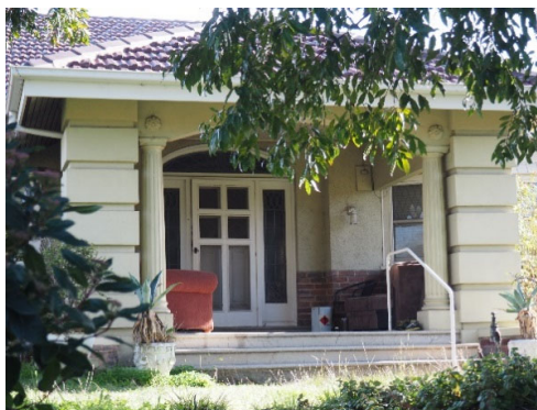
Figure 6. The central entry to the building features glazed sidelights and a shallow arched fanlight. The portico employs classical details. (Source: Trethowan Architecture 2018)
