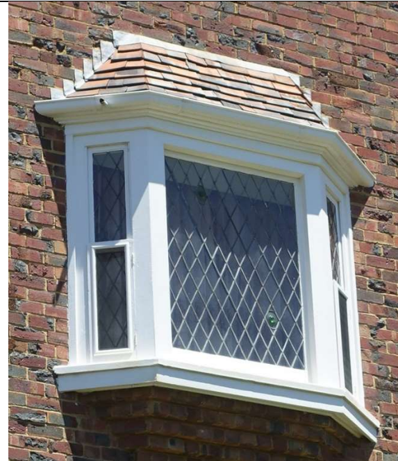
Oriel window of first floor. Note diamond leadlights with coloured bullseye accents, and terracotta shingle roof.
