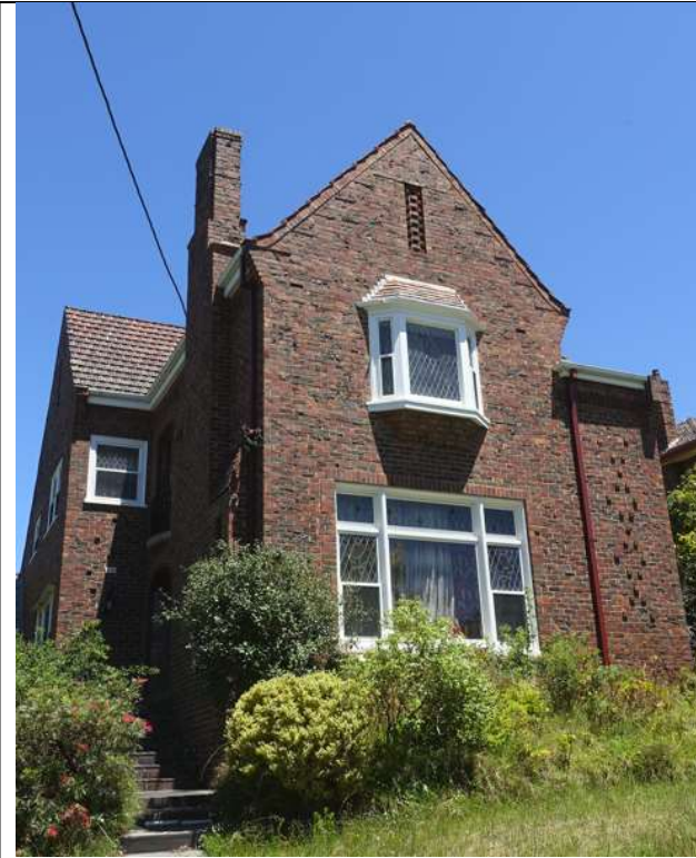
Oriel window of first floor. Note diamond leadlights with coloured bullseye accents, and terracotta shingle roof.
