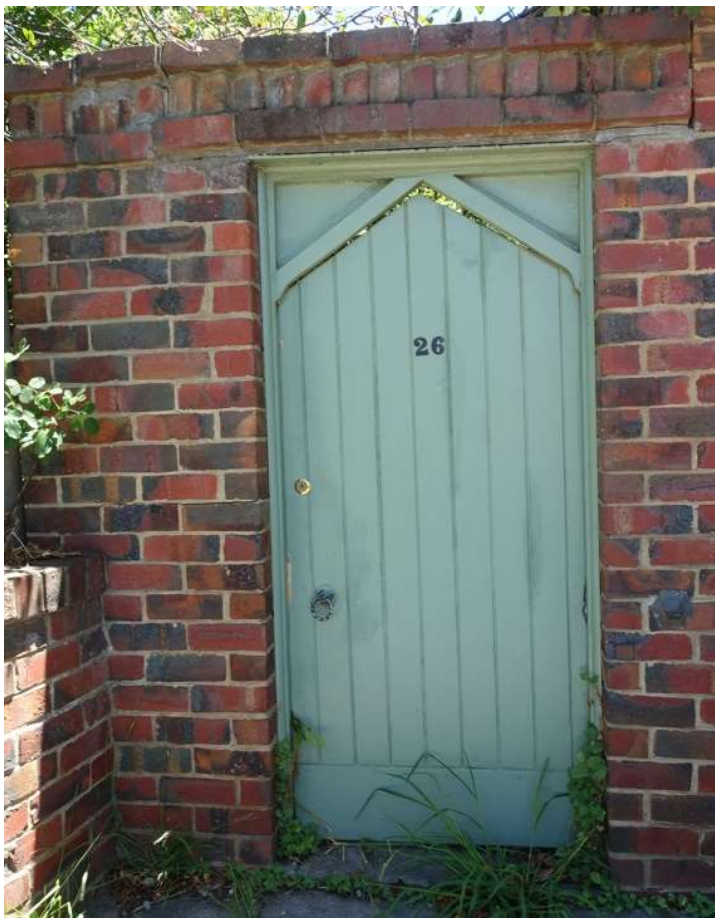
Figure 10. The brick fence adjacent to the garage. Note the movement of bricks in the parapet and some inexpert repointing. (GML, 2022)
