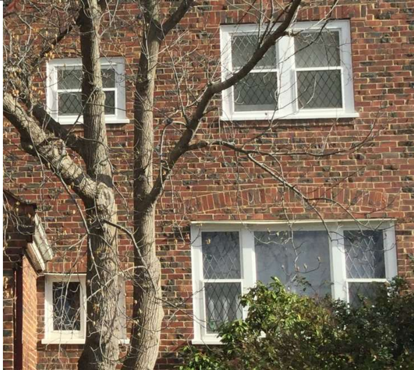
All windows retain the diamond leadlights as on the plans. The Chicago window at lower right incorporates coloured bulleyes (2017).
