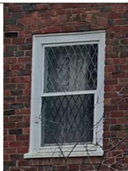
An intact first-floor windows with two diamond light sashes (2020). Only the upper sash was visible in January 2022; it was intact.
