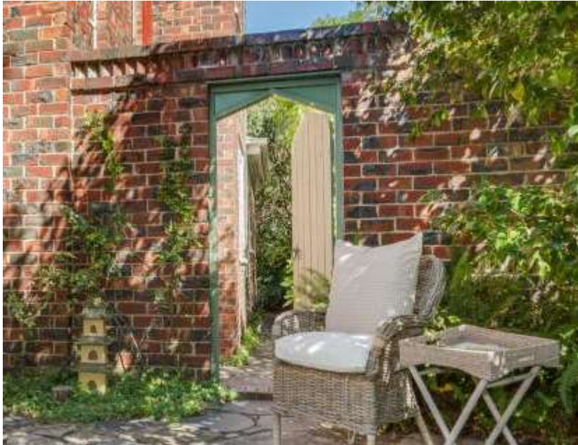
Figure 11. Wing wall/brick fence on the western side of the house. Note grey (re-)pointing above the gateway. ( https://www.realestate.com.au/sold/property-house-vic-kew-119529784 , 2015)
