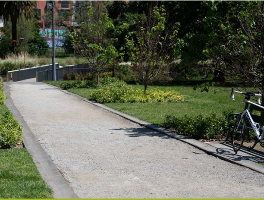
Minimum 3m wide path with unsealed surface and concrete edging to prevent path washout
