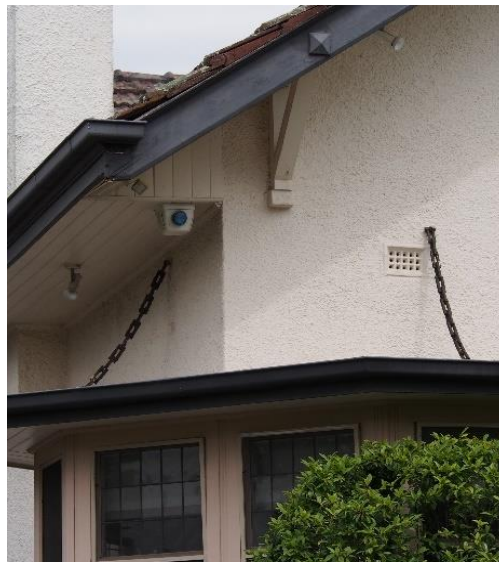
Figure 8: Chains to flat roof of corner bay window. Timber struts support the projecting gable end above. (Source: Trethowan Architecture, 2017)
