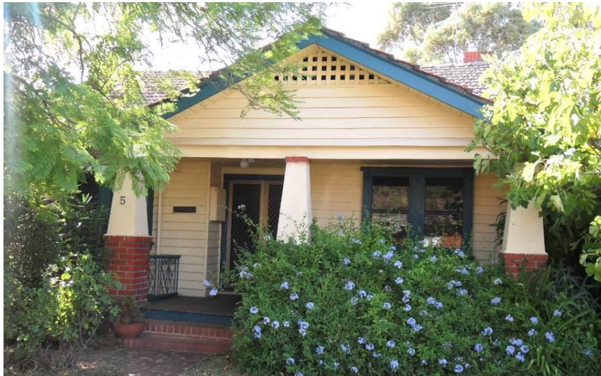
Figure 18. Timber California Bungalow with a transverse gabled roof and gabled porch on tapered piers at 5 Munro Street, Hawthorn East. (Source: Context, 2018)
