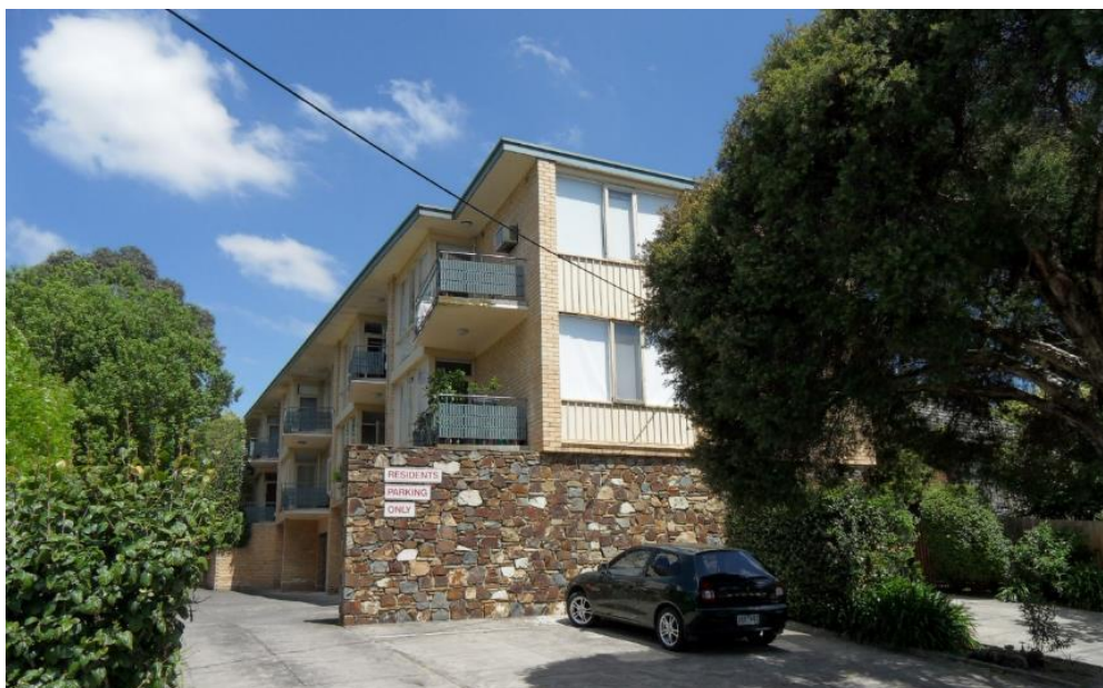
Figure 6. View of the principal elevations of the building (facing south-west from Denmark Hill Road). Note the cantilevered massing of the upper floors above the feature stone wall. The splayed balconies run the depth of the east elevation. The wall-mounted air conditioning unit visible at second-floor level is a later addition. (Source: Trethowan Architecture, 2017)
