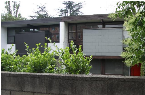
Figure 10. View of 406B & C. Note the original details to 406B, including the double hung timber sash windows, with fixed glazing below (Source: Trethowan Architecture, 2017).
