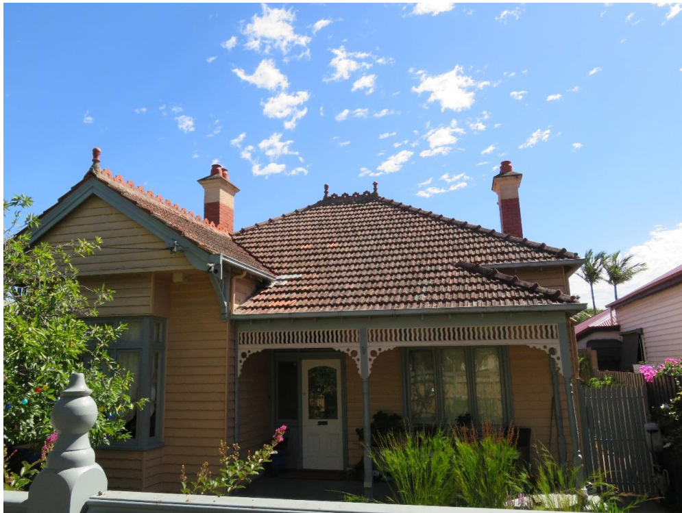
Figure 13. Timber Edwardian house with weatherboards at 17 Harts Parade, Hawthorn East. The verandah detailing, including the timber fretwork is distinct from that of the earlier Victorian era houses in the precinct. (Source: Context, 2018)
