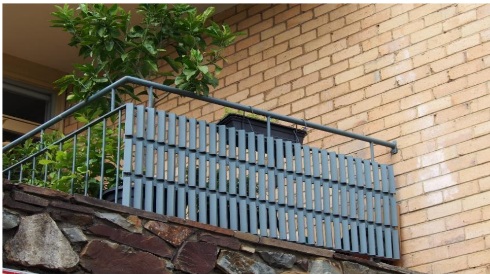
Figure 8. Detail view of typical balustrade detail (Note the right-angle steel work screen, welded to a standard balustrade that provides additional screening) (Source: Trethowan Architecture, 2017).
