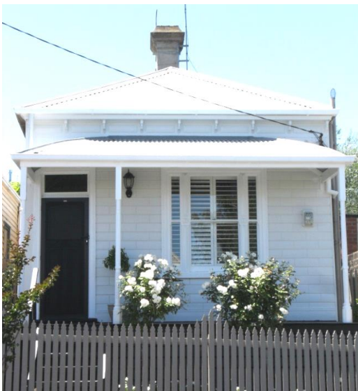
Figure 9. One of the timber houses with the small-scale timber ashlar at 27 Oberon Avenue, Hawthorn East, which also retains its original verandah columns (missing their capitals). (Source: Context 2018)
