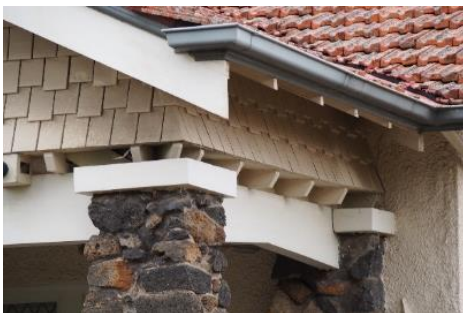
Figure 4. Shingles wrap the porch, supported by visible timber framing and tapered bluestone columns with squared-off capping. (Source: Trethowan Architecture, 2017)
