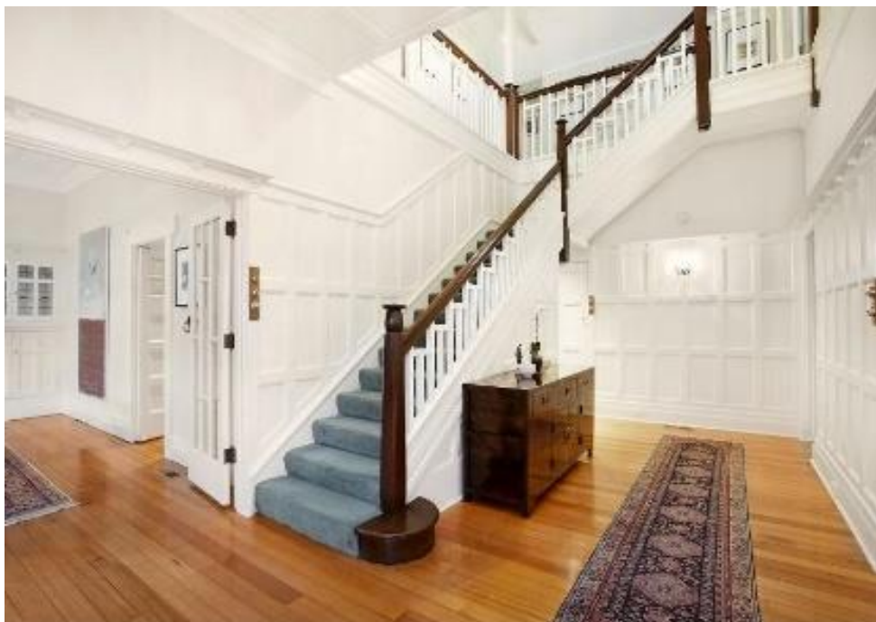
Figure 9. Original interior features have been retained, including wainscoting, stair and balustrade, architraves and doors, and decorative ceilings, although the colour scheme has been painted over. (Source: realestate.com.au, 2016)
