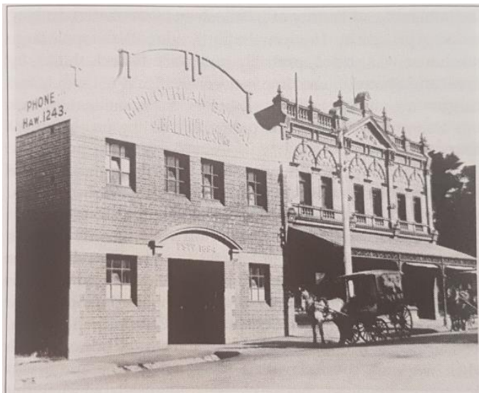
Figure 5. Balloch's bakery pictured c.1920, with loading bay off Auburn Road. Note the quoins, entry and window openings which are incorporated into the current façade. (Source: McFarlane 1992:33)
