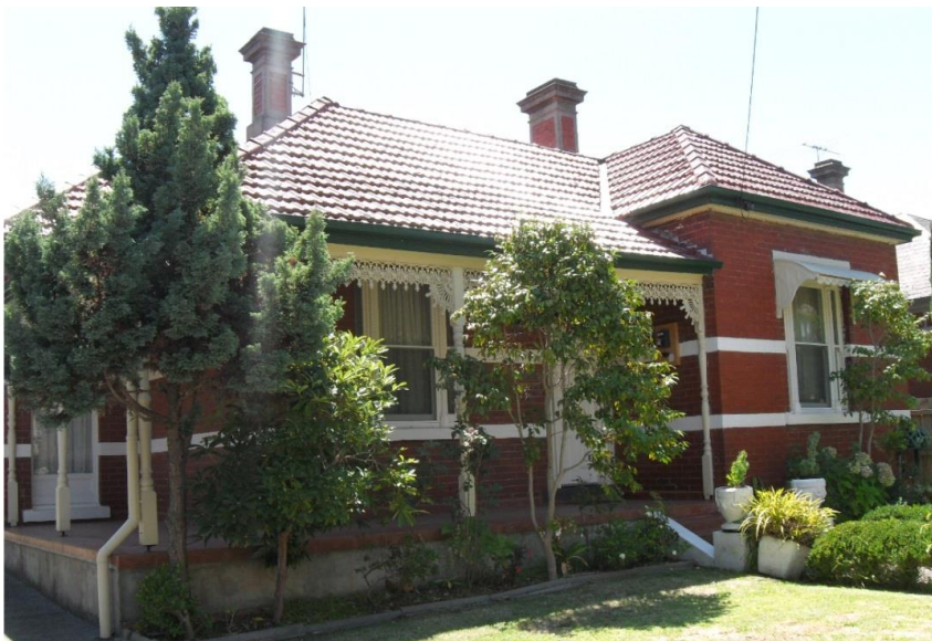
Figure 7. A c1901-03 Italianate house at 29 Harold Street. Note the use of red face brick, turned timber posts and a pressed-metal window hood, all indicative of its twentieth century date. (Source: Context, 2018)
