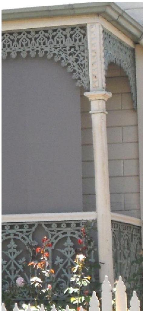
Figure 10. The verandah at 25 Oberon Avenue, Hawthorn East, with original stop-chamfered posts, cast-iron frieze, brackets and balustrade. (Source: Context 2018)
