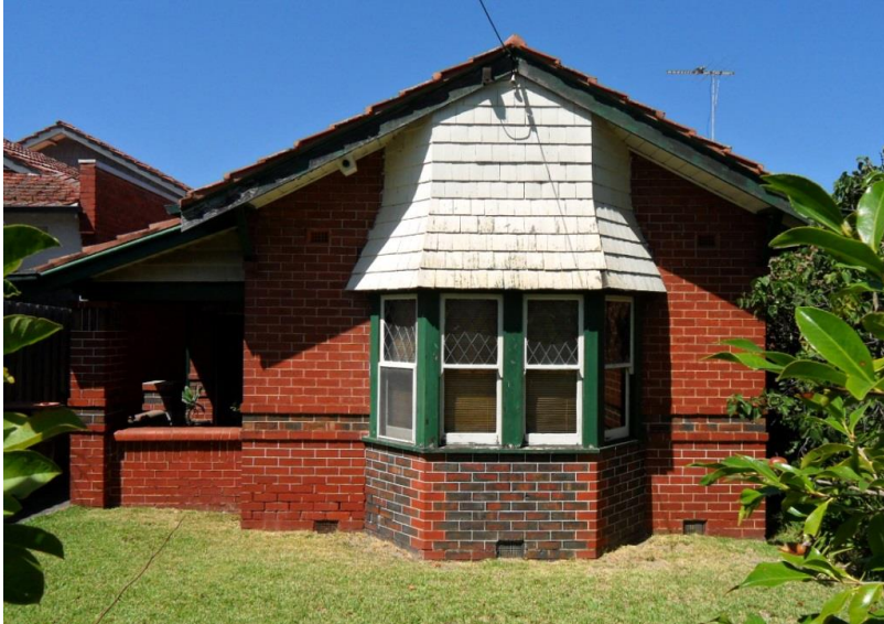
Figure 17. California Bungalow at 746 Burwood Road with hipped-gable and gabled roof forms. Note the shingled hood to the front bay window. (Source: Context 2018)
