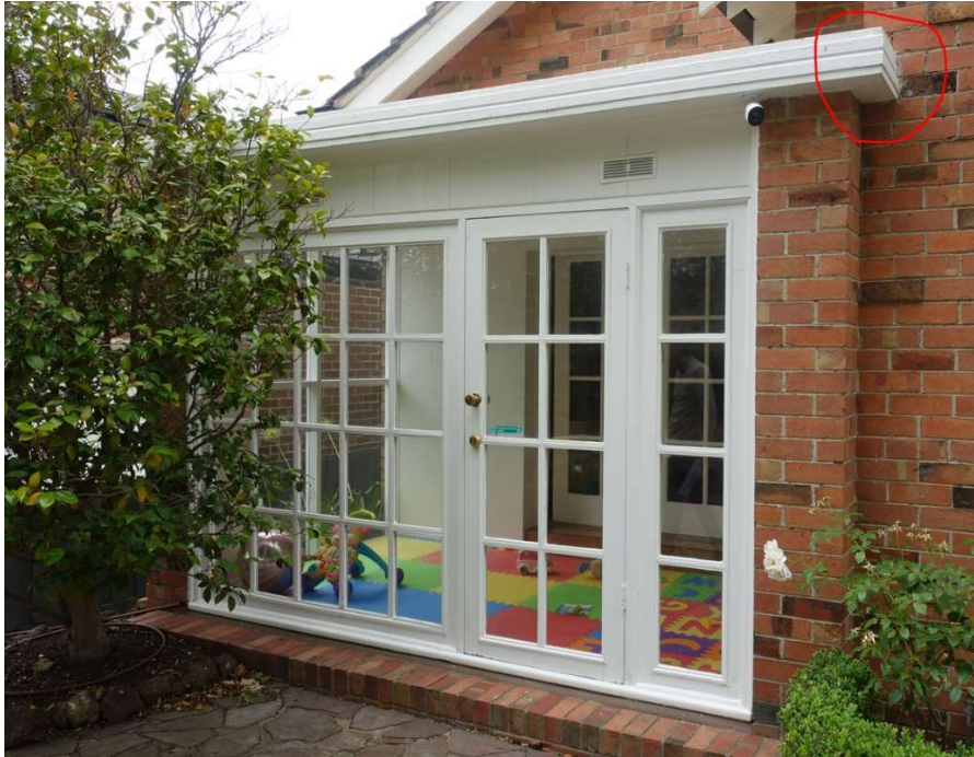
Figure 93. 60 Hortense Street sunporch. Note the concrete roof slab, with incised horizontal lines from a formwork mould, which is let into the wall at the north end (circled). Note also the use of the same bricks for the pier (at right) and floor of the sunporch as the rest of the front façade. The original French doors are visible inside the sunporch. (Source: Context, 2019)
