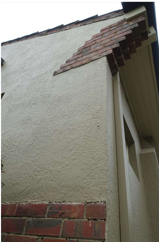
Figure 32. South corner of the front façade, showing brick accents that are still proud of the render. (Source: Context, 2019)
