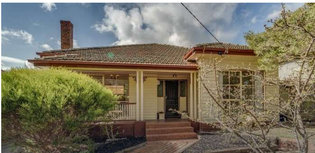
Figure 18. 41 Fairview Avenue, Camberwell, a contributory property in HO225 Fairview Avenue Precinct. The front windows of this 1930s timber bungalow have been replaced and enlarged, the porch supports replaced and neo-Federation fretwork installed. (Source: Domain.com.au, 2021)
