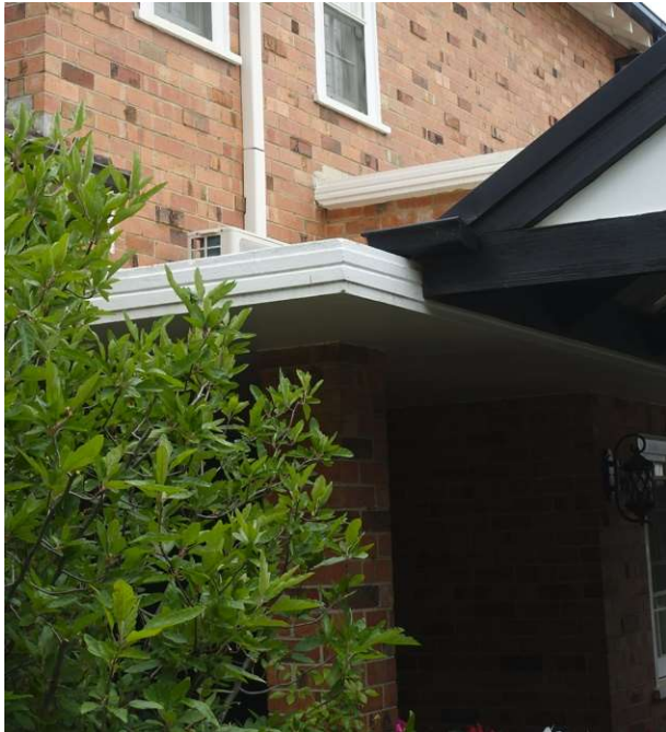
Figure 95. Detail of the front entry on the north side of the house. Note the same concrete slab profile, with incised horizontal lines, as seen on the sunporch, indicating that it was created with the same formwork mould. (Source: Context, 2019)
