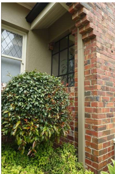
Figure 31. North side of the front porch, with infilled original opening. (Source: Context, 2019)
