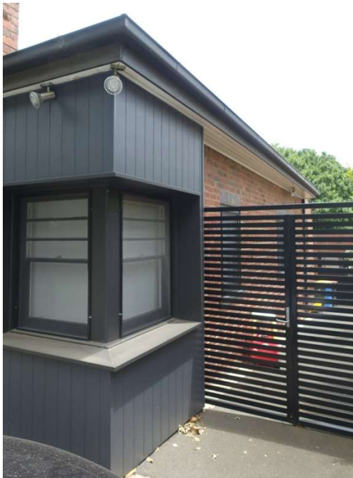
Figure 63. North-east corner of 56 Florizel Street, with the return of the new cladding extending as far as the corner window. (Source: Context, 2019)
