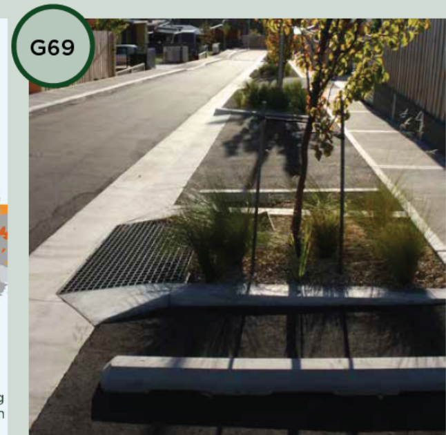
Figure 27: Storm water runoff from carparks is to be collected and redirected to passively irrigate trees - Maroni Close, Berriedale (Urban Initiatives)
