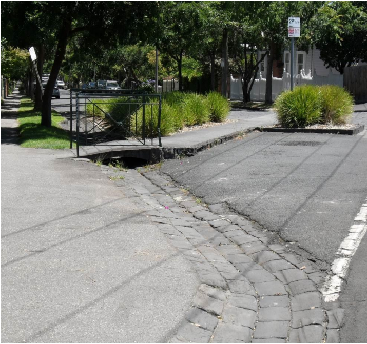
Figure 5. Bluestone pitched channel which runs along the west side of the railway line (Newport Crescent and 48-68 Auburn Parade). Note that the footbridge is modern. (Source: Context 2018)
