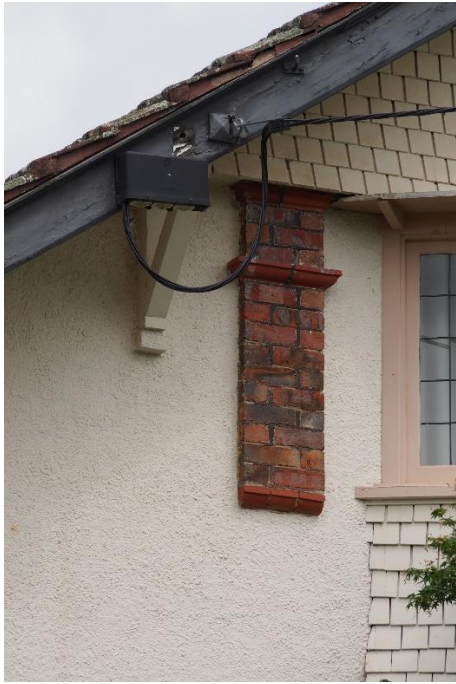
Figure 3. Engaged red brick pilasters by oriel bay window. (Source: Trethowan Architecture, 2017)
