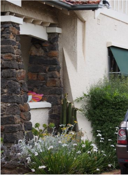
Figure 2. The north-west corner of the house as a deep, roughcast buttress. (Source: Trethowan Architecture, 2017)
