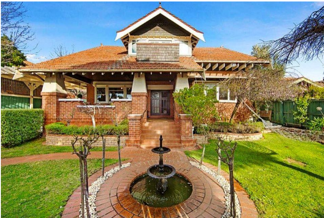
Figure 8. Perspective of the primary elevation of the subject property. Note the box framed window under the verandah, the varying rafter types depending on position and the stepped balustrade capping of the verandah. Not visible, but adjacent to the door is a name plaque bearing 'Les Cloches'. (Source: Domain.com)
