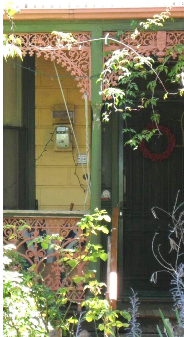
Figure 11. The verandah at 10 Tara Street, Hawthorn East, with original round tapered posts (capital missing), cast-iron frieze, brackets and balustrade. (Source: Context 2018)
