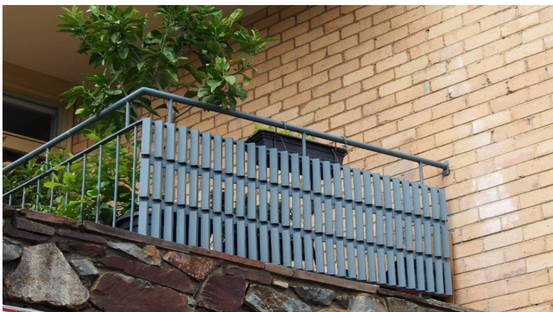
Figure 8. Detail view of typical balustrade detail (Note the right-angle steel work screen, welded to a standard balustrade that provides additional screening) (Source: Trethowan Architecture, 2017).
