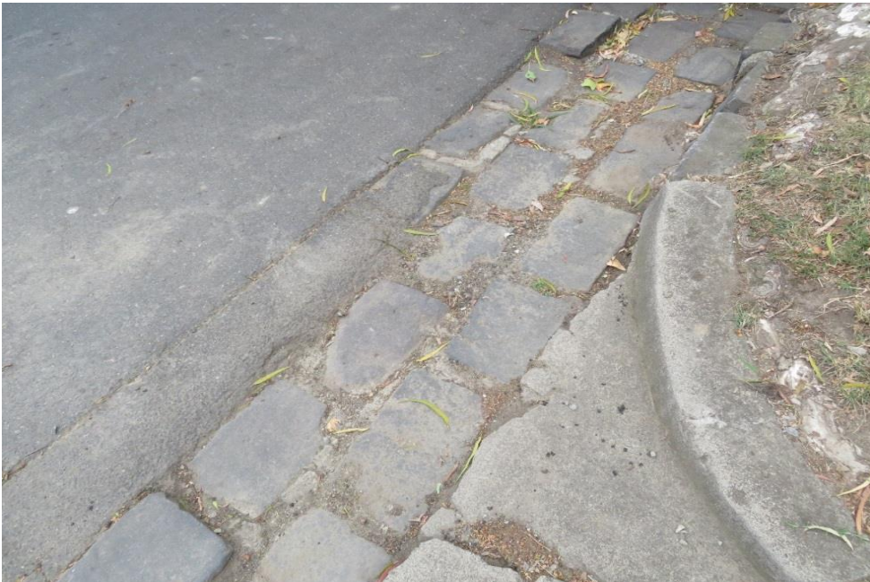
Figure 8. Bluestone guttering remaining in situ along the north and south sides of Currajong Road. (Source: Context, 2018)
