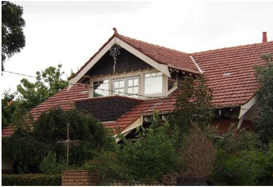
Figure 6. View of the upper portion of the dwelling from the west. Note the terracotta horn finials and chimney cowls. Also visible is the cut-away of the roof and taper cut bargeboards. (Source: Trethowan Architecture, 2017)
