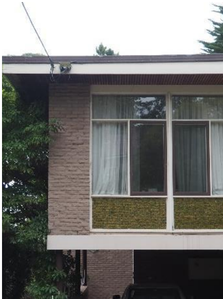
Figure 10. View of the window and walling detail. Note the small green mosaic tiles and the rough brick walling. (Source: Trethowan Architecture, 2017)
