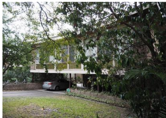
Figure 9. View across the façade from the east of the site. Note the low wall down the driveway and the raised garden bed below the line of the façade, elements from which the pilotis rise. (Source: Trethowan Architecture, 2017)
