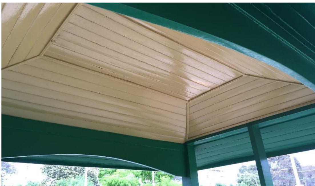
Figure 11. Internal view of the shelter, showing the vaulted tongued and groove lined ceiling and eaves. Note the simple timber arch which extends between the vertical posts at north and south ends of the structure. (Source: Trethowan, 2017)
