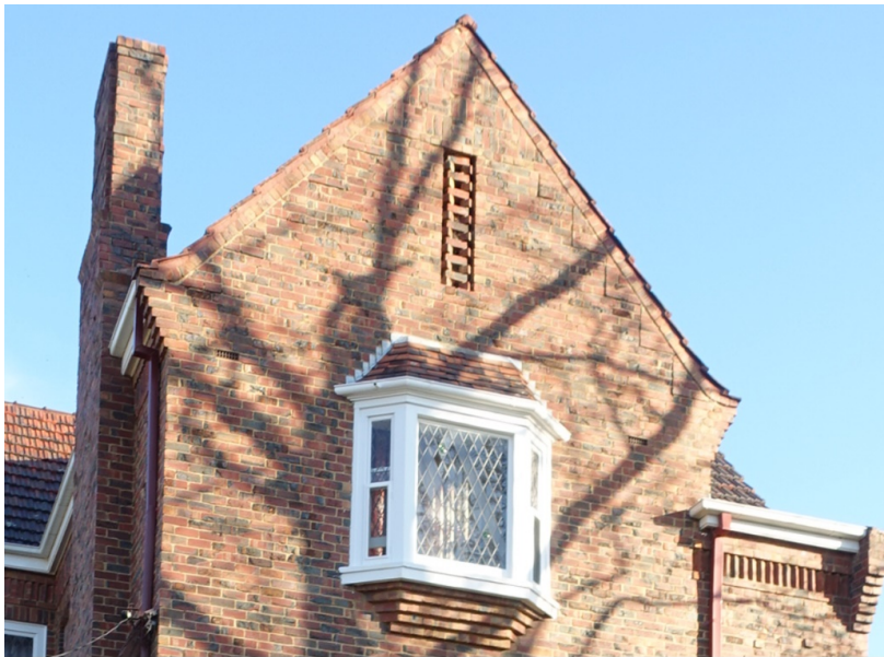
Figure 6. Brickwork details to the front façade, including herringbone pattern and quoins to the gable, vent, corbelling below the oriel window, and the ribbed eaves detail. (Source: Context, 2019)
