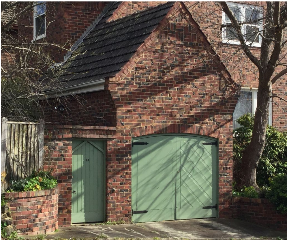
Figure 8. Attached garage and back gate. Note brick detailing to garage gable and timber garage doors, ledge door to back yard in brick surround. (Source: Context, 2017)
