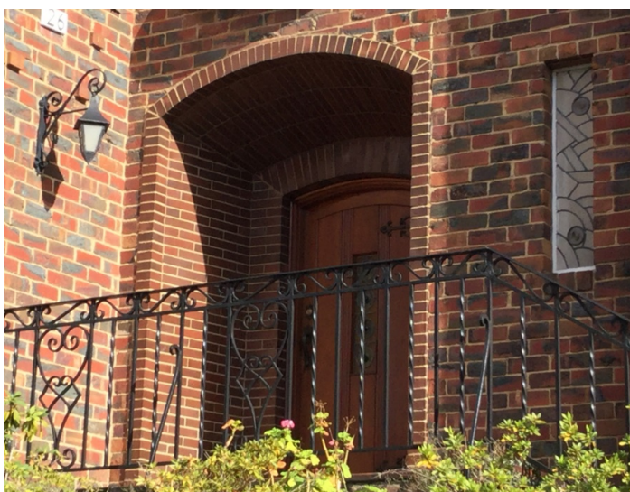
Figure 7. Detail of the front entrance, including a lantern, the linen-fold door with strap hinges, mild-steel balustrade, and abstract leadlight window. (Source: Context, 2017)
