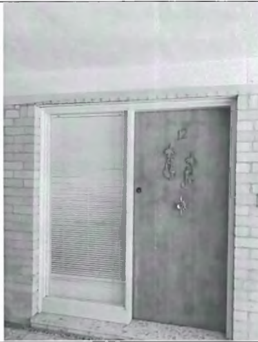
Front door with original stain finish and applied decoration. Note also the nougat terrazzo floor finish
