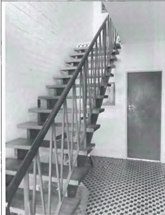
Open treads and tiled pavement floor with simple decorative metal balustrading of the period.
