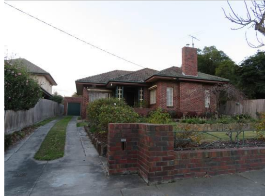
Figure 25. 15 Macdonald Street. Brick fence with mild-steel panels between piers. (Source: Context 2018)
