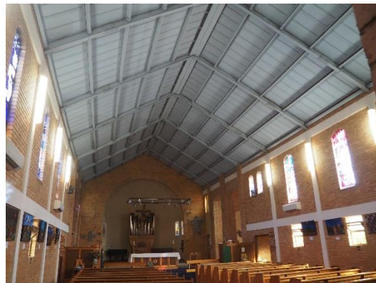
Figure 11. Interior view of the Church. Note the cream brick walls and expressed portal frame structure. (Source: Trethowan Architecture, 2018)
