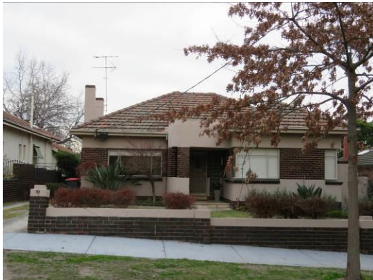
Figure 26. 10 Faircroft Avenue (HO43) fence of brick with rendered upper course matching details of the house. (Source: Context 2018)
