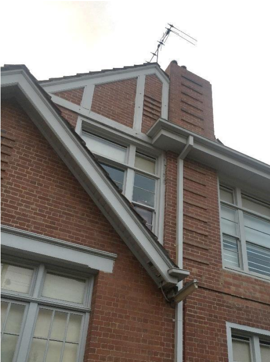
Figure 15. Detail of the 1947 upper level gable intersecting with the brick chimney. (Source: Context, July 2018)
