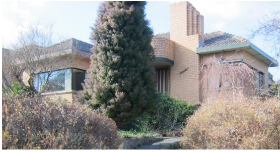
Figure 24. Late interwar Moderne house of 1940 at 67 Brandon Street. Note the cream brick, steel windows, and stepped chimney. (Source: Context 2018)
