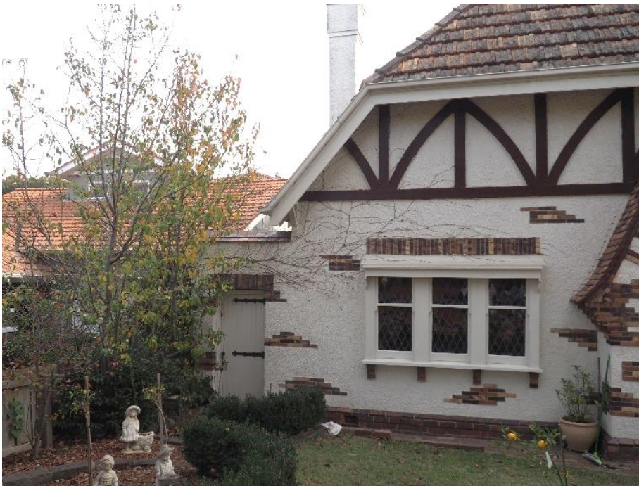
Figure 6. Detailing of brickwork, framing and half timbering around window (Source: Trethowan Architecture, 2018).
