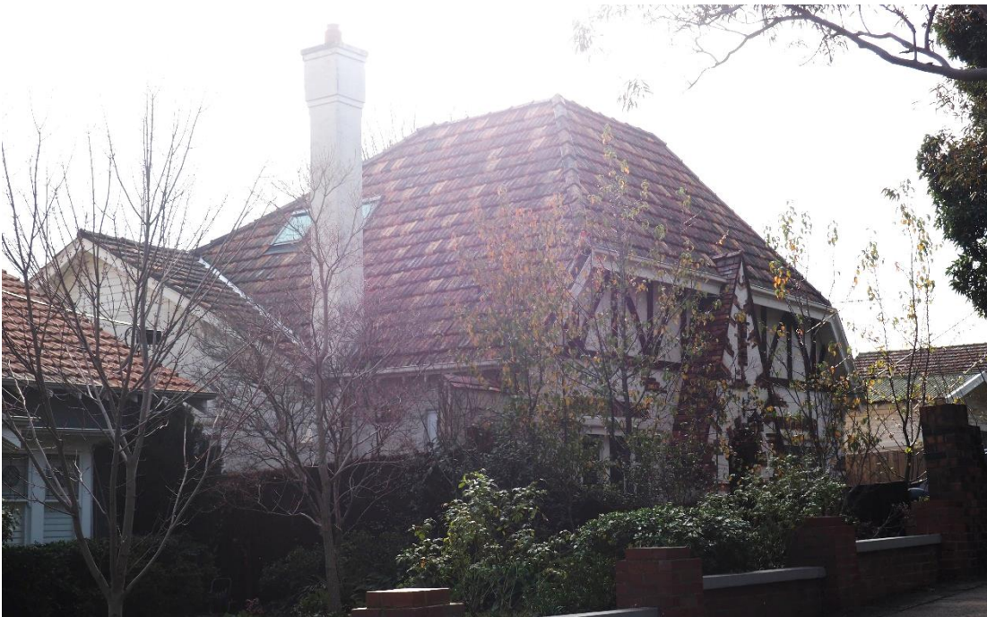
Figure 10. View of the unusual roofscape at 2 Allison Avenue. Note the front portion emerges steeply from the transverse gable behind. (Source: Trethowan Architecture 2018)
