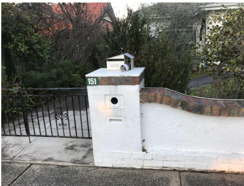
Figure 21. Original rendered and brick front fence with mild-steel gates to 151 Glen Iris Road. (Source: Context 2018)
