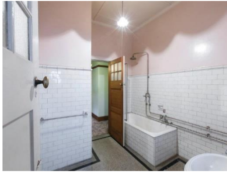
Figure 8. The bathroom includes original fittings and finishes, such as surface mounted plumbing, wall tiles, terrazzo flooring and original doors and door hardware. (Source: Marshall White Real Estate 2015)
