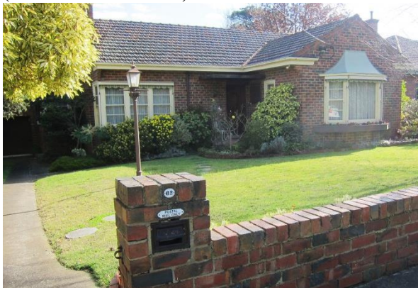
Figure 17. Early post-war Old English house at 62 Brandon Street (1948). Note the clinker brick, canted bay window with bell-cast eaves, low gable slope and corner window. (Source: Context 2018)
