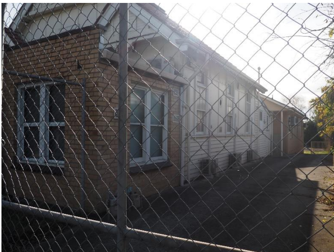
Figure 13. View down the eastern elevation of the former timber chapel. Note the lead-lighting to above the sash windows, and half weather-boarding to the elevations. (Source: Trethowan Architecture 2018)
