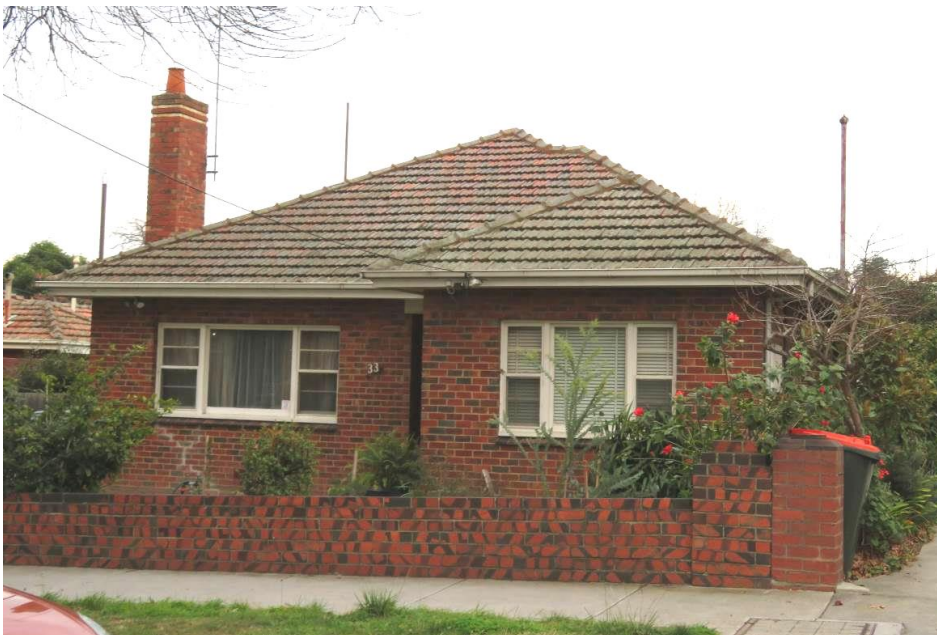
Figure 18. The early post-war house (1946) at 33 Rix Street. Note the clinker brick walls, projecting hipped bay, and horizontal window glazing bars. (Source: Context 2018)
