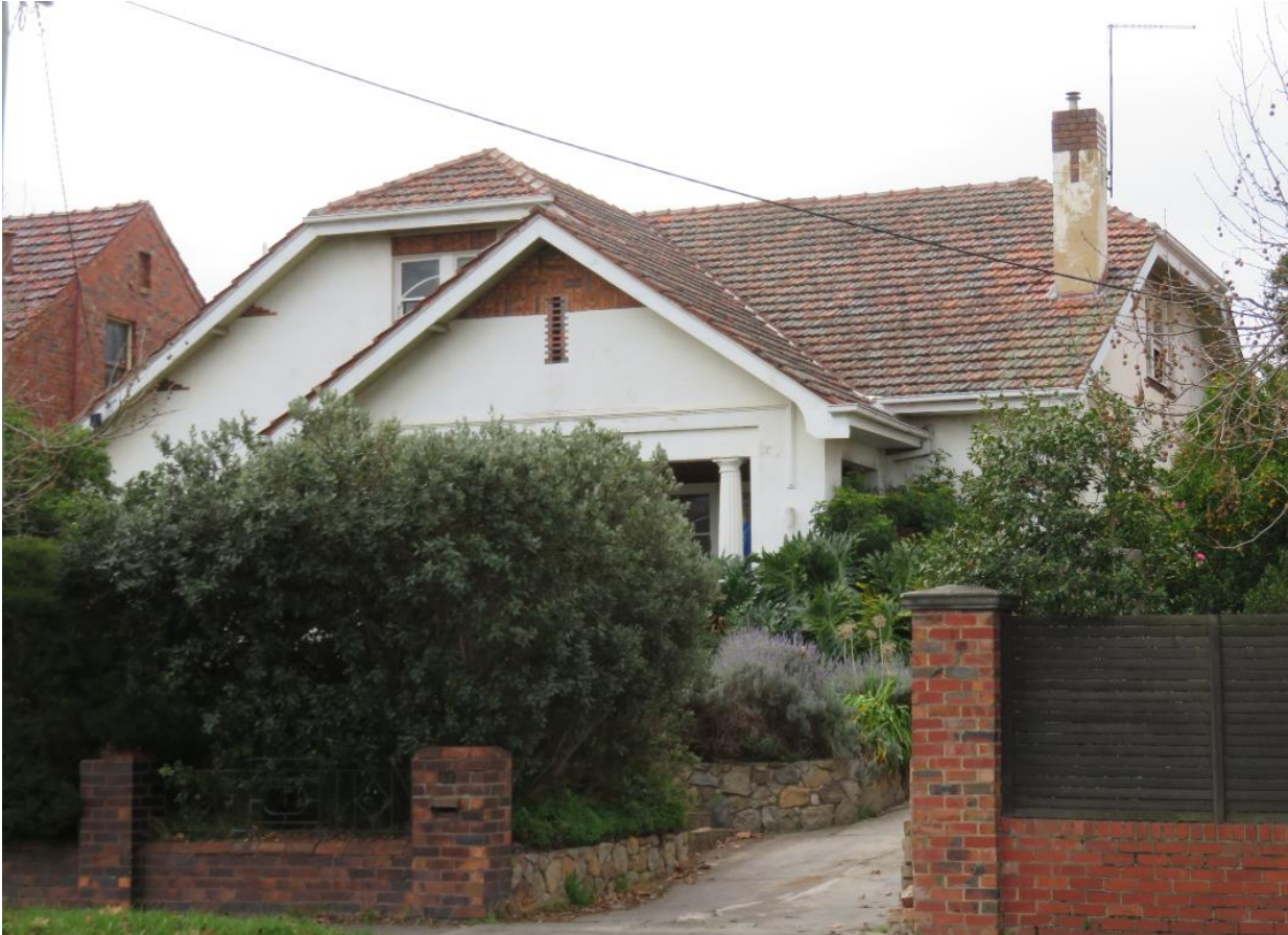
Figure 15. A picturesque example of the Old English style at 139 High Street incorporating rendered walls with tapestry brick accents and jerkin-head gables, of 1935. (Source: Context 2018)
