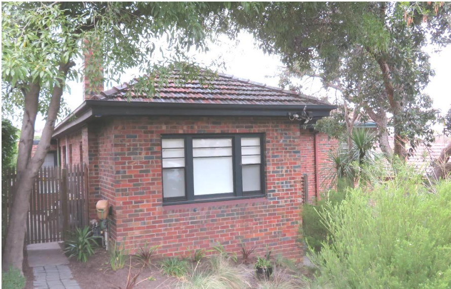
Figure 17. The late interwar dwelling at 7 Parkin Street (1941). Note the clinker brick walls, projecting hipped bay, and horizontal window glazing bars. (Source: Context 2018)
