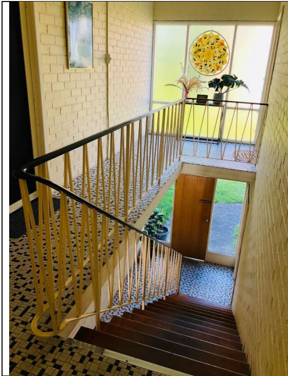
Mosaic Tiling to upper and lower levels in common stairwells.
