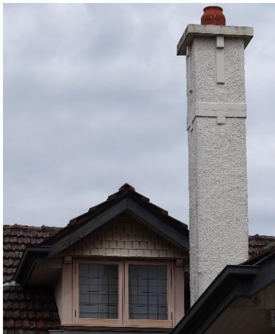
Figure 4. Chimney with decorative capping treatment. (Source: Trethowan Architecture, 2017)
