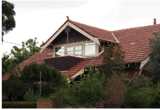
Figure 6. View of the upper portion of the dwelling from the west. Note the terracotta horn finials and chimney cowl. Also visible is the cut-away of the roof and taper cut bargeboards. (Source: Trethowan Architecture, 2017)
