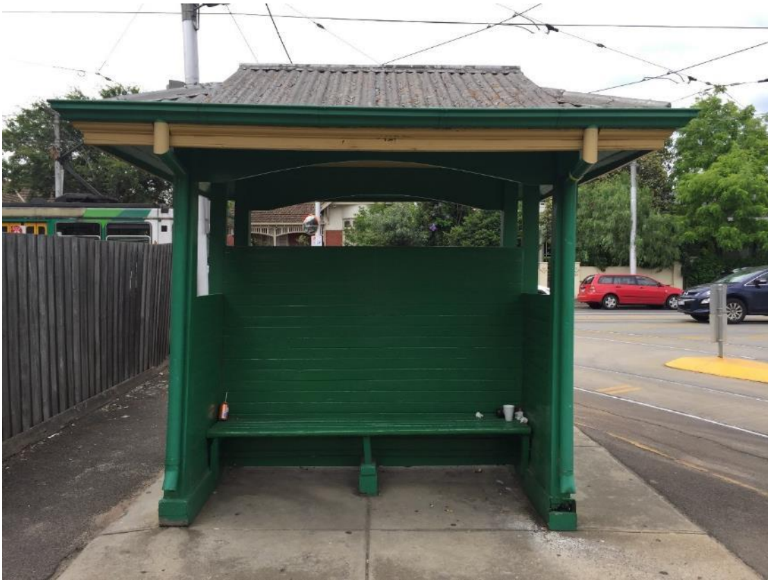
Figure 10. View of the north elevation of the tram shelter. Note the height of the weather shields to the left and right of the back rest at the centre of the structure and the timber arches either end of the structure. At right of the image, rot to the bottom of the post and plinth is evident. (Source: Trethowan, 2017)
