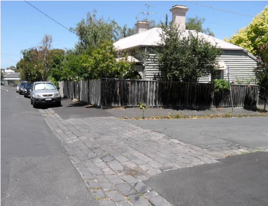
Figure 4. Intersection of Oberon Avenue and Tara Street, looking south. Note the wide bluestone channel without a kerb to Oberon Avenue (widening at the intersection), and the more standard bluestone kerbs and narrow channel on Tara Street. (Source: Context 2018)
