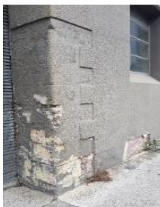
Figure 15. Detail of the original quoined corners with stone and brick underneath. (Source: Trethowan Architecture, 2018)
