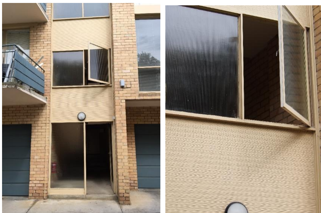
Figure 10. View of the main entrance on the east elevation, facing the car court (Note the original ribbed glazing and textured Masonite spandrel panels). The garage doors either side are also original features. (Source: Trethowan Architecture, 2017)
