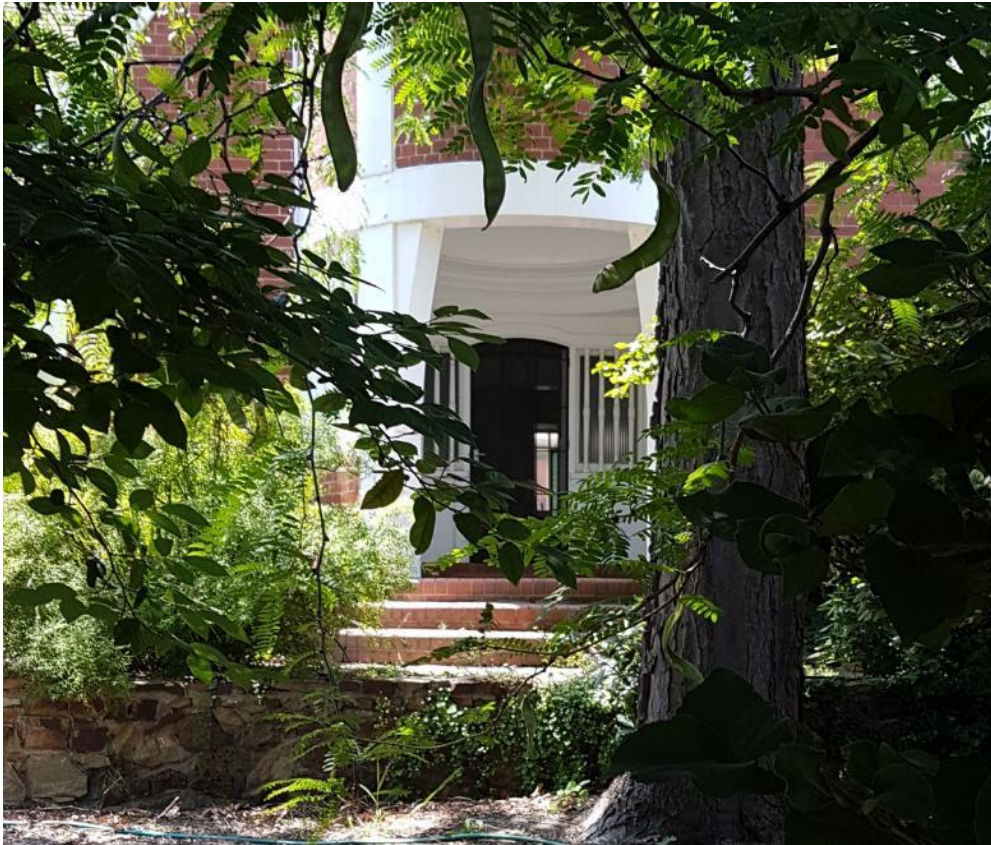
Figure 12. View of the front porch showing intact steps, porch entry pilasters and doorway, porch ceiling, and balusters. (Source: Trethowan Architecture, 2018)
