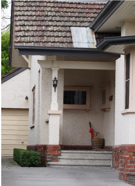
Figure 7. Entry porch with timber framing, original terrazzo steps and landing, and box-framed windows. (Source: Trethowan Architecture, 2017)
