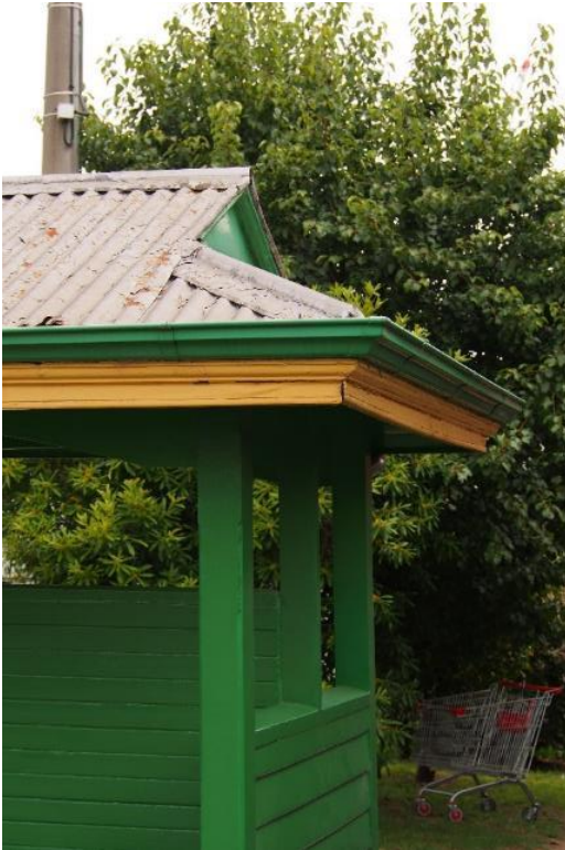
Figure 12. View of the south-east corner of the tram shelter, showing the beaded barge boards with supporting timber ovolo moulding to the underside of the ogee guttering. Note the silver painted finish to the corrugated sheet metal roofing, exposing rust to the bare metal sheet beneath. (Source: Trethowan, 2017)
