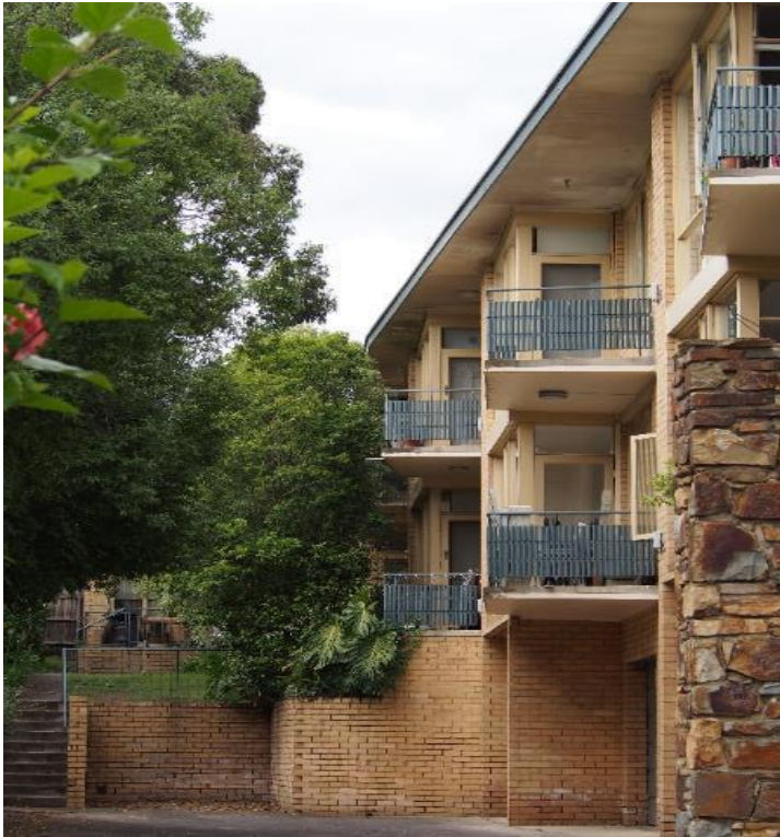
Figure 7. View of the principal east elevation (facing south-west from the internal driveway). Note bespoke steel work balustrading and added detailing to the north face of the balustrade providing additional privacy from views from Denmark Hill Road. (Source: Trethowan Architecture, 2017)
