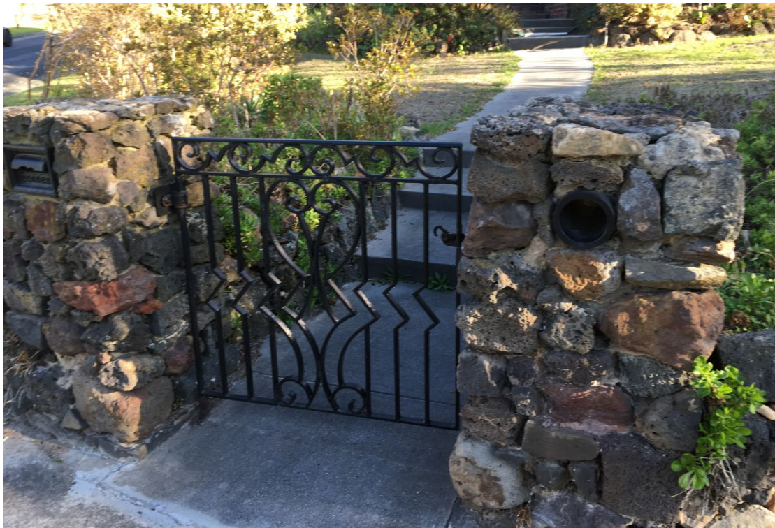
Figure 4. Detail of the front gate and associated rubble stone piers. (Source: Context, 2019)
