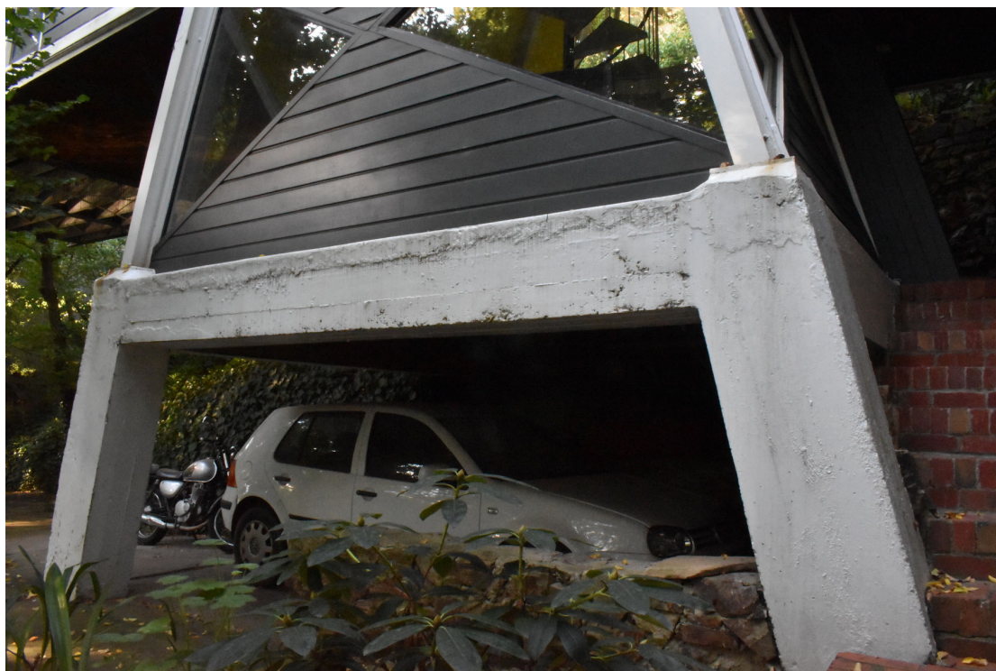
Figure 8. Concrete plinth.
