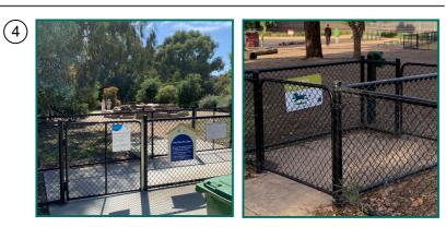
1.5m high post & wire fencing around perimeter of fenced dog play area
