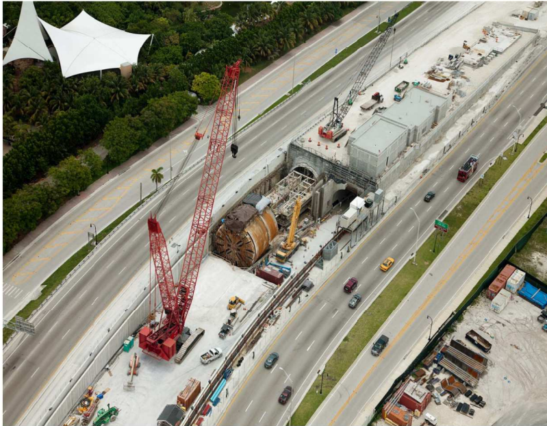
Figure 19: Example of a TBM disassembly in a congested situation
