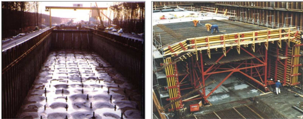
Figure 2: Construction of Cut & Cover tunnelling
